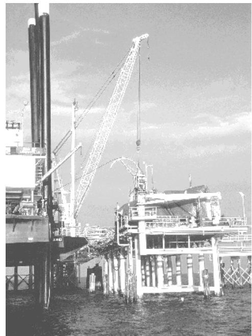
Figure 19. Offshore CT Operation
