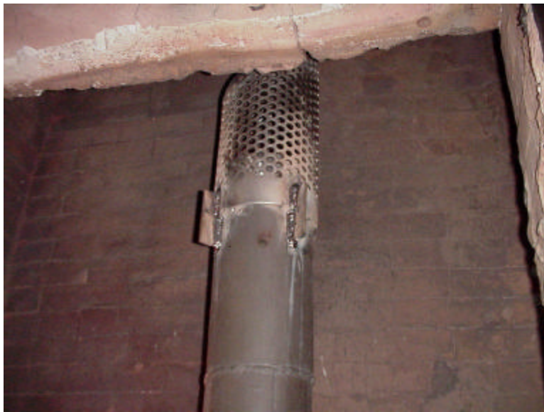
Figure 5.4-11: Perforated Grizzly Design
