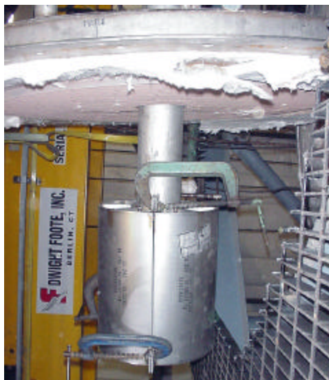
Figure 5.2-3: Bauxite Distributor Being Mounted To Roof
