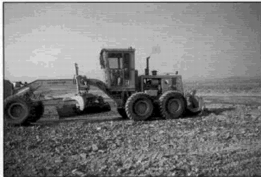
Figure 3-8. Road grader ripping a site during site preparation.
