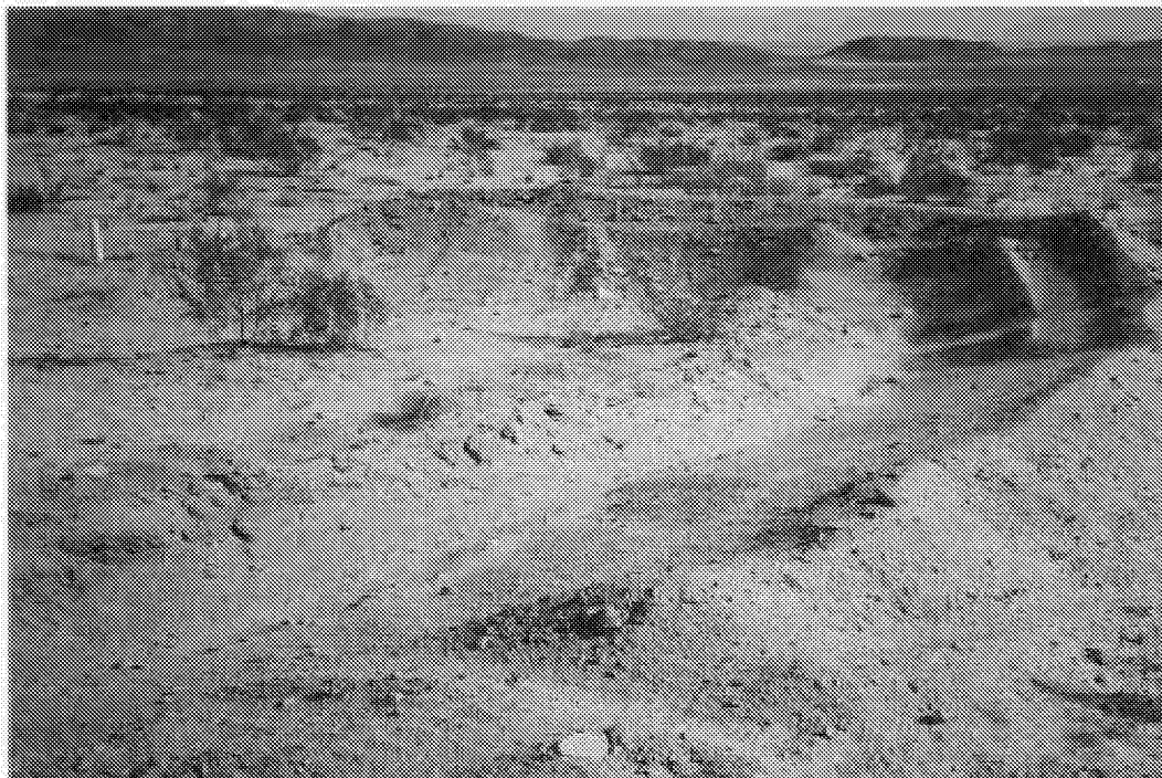
Figure 3-4. Dozer basin used to catch runoff from roadway and upslope in Fort Irwin, California.
