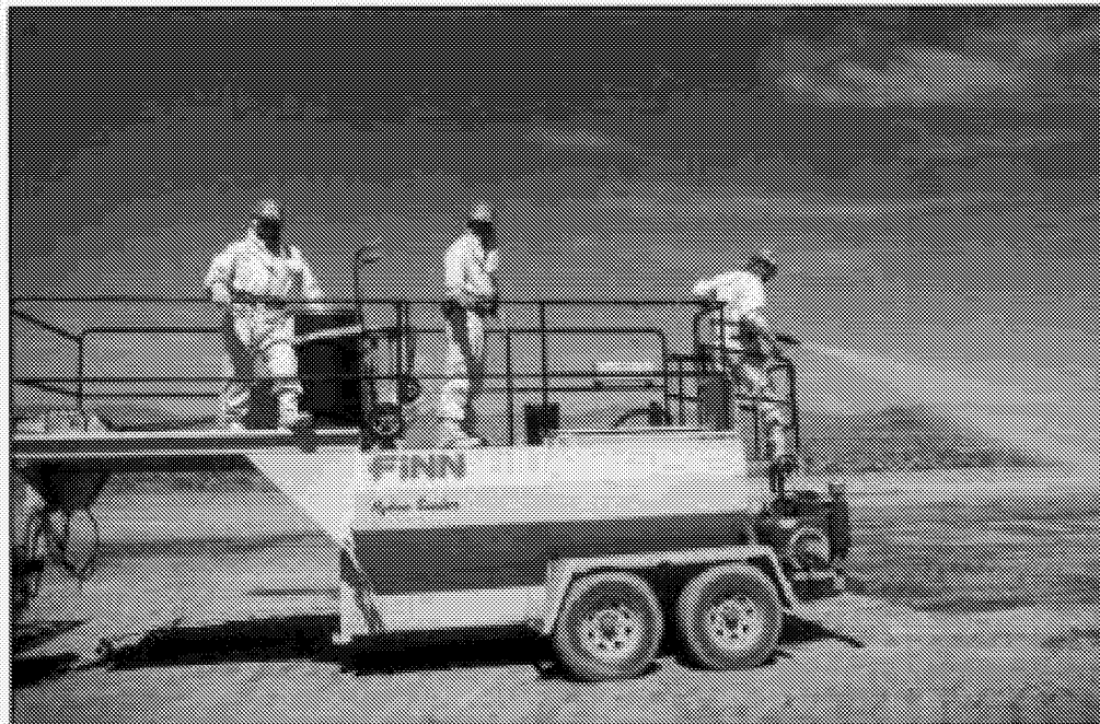
Figure 3-6. Applying chemical soil stabilizer with a hydromulcher.
