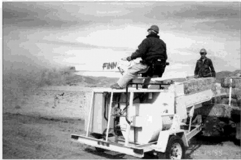
Figure 3-27. Applying straw with a blower requires three people.
