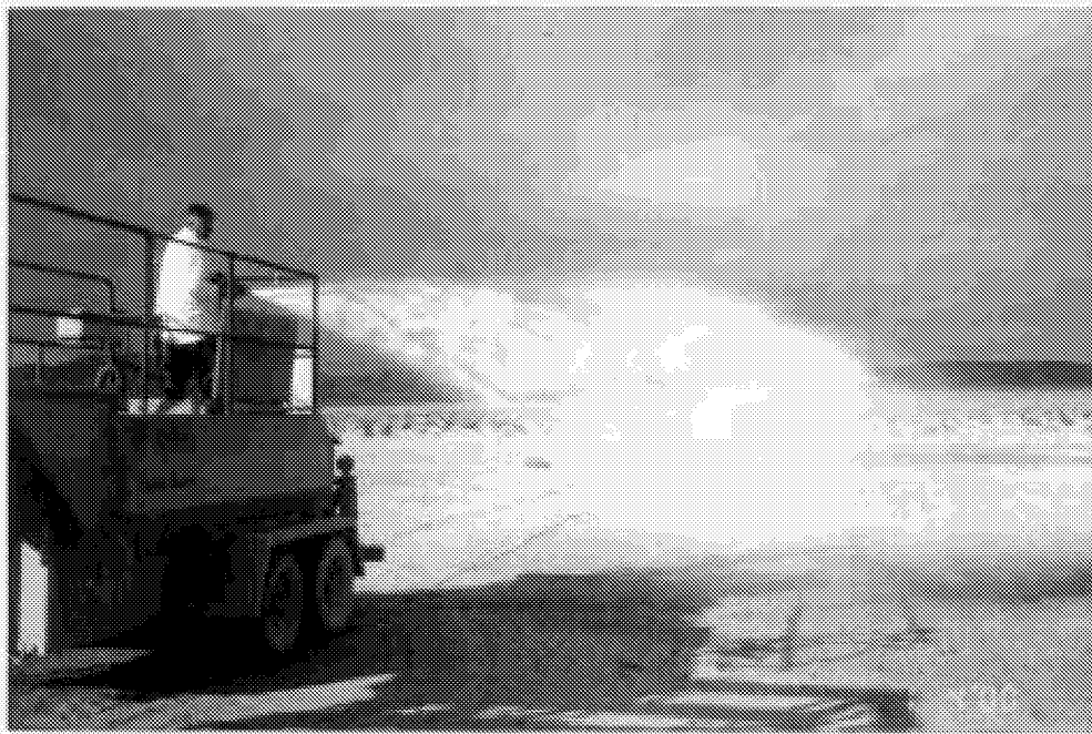
Figure 3-29. Applying tackifier with a hydroseeder.
