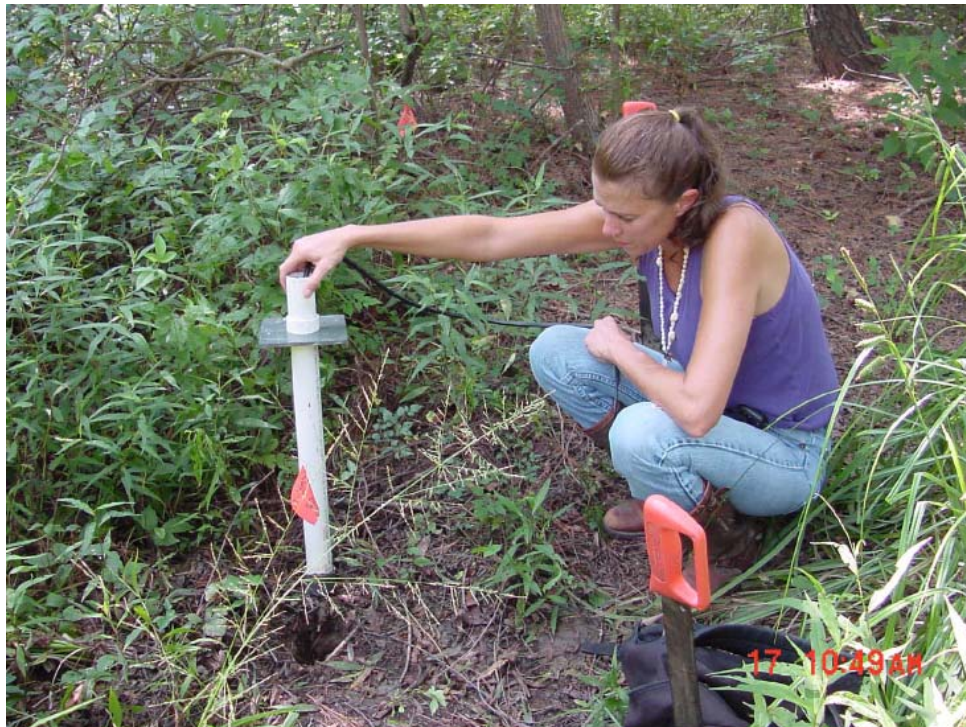
Photo 2. Inserting the Pipe into the Bore Hole
