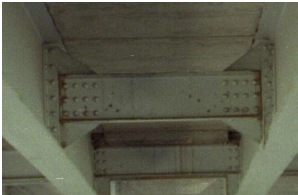
Figure 5. Photo of interior cross braces.
