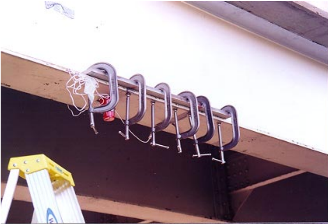
Figure 70. Clamps and plate used to stiffen the structure locally.
