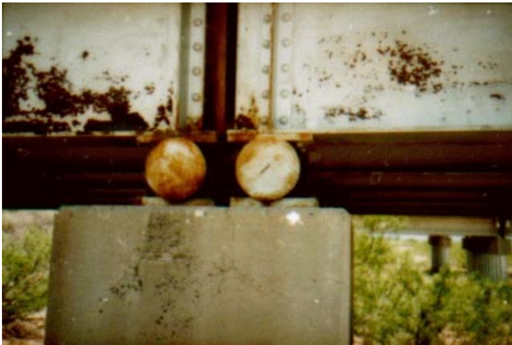
Figure 9. Roller connections at the northern-most pier.
