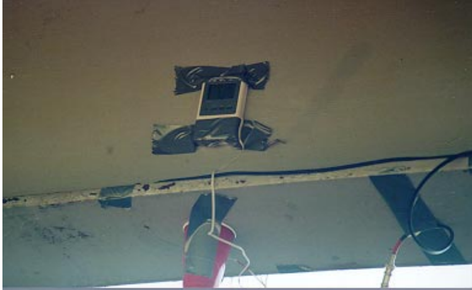
Figure 34. Indoor-outdoor thermometer taped to the exterior girders.
