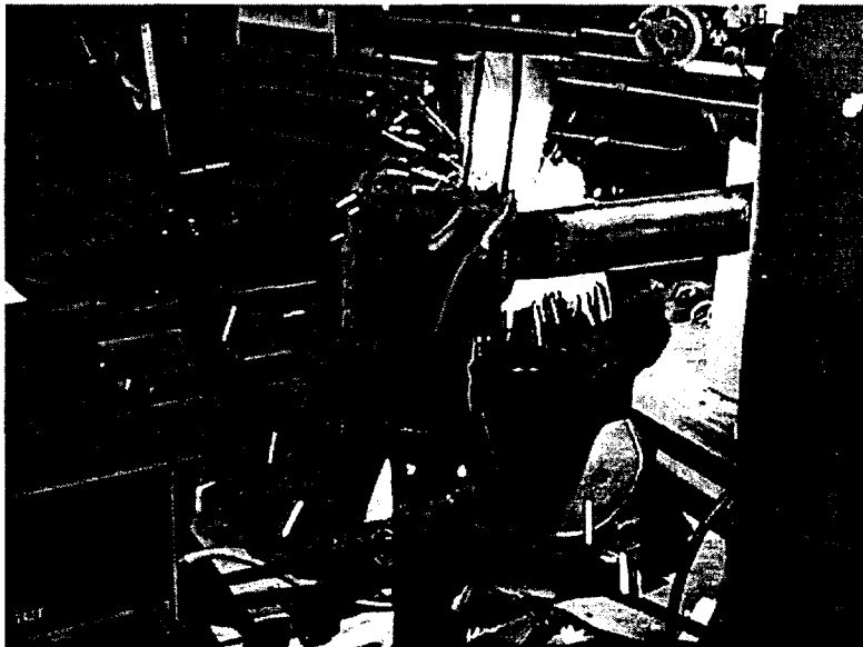
Figure 2. Welding of the replaced horizontal section of the melter . The replacement reverted the vertical orientation of the pour spout.
