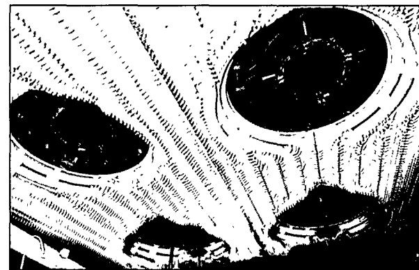
▲ The Babcock & Wilcox Company DRB-XCL ® burners, installed on a down-fired boiler, were used in the Integrated Dry NO x /SO 2 Emissions Control System project.
