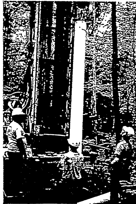
A casing is prepared for lowering into a borehole.
