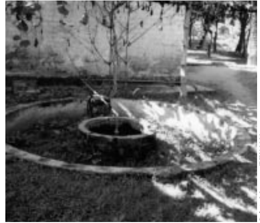
Figure 6.9. Biogas plant digester.
