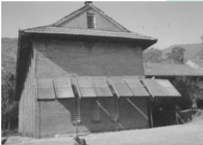
Figure 2.7. This solar water heater has provided hot water to this school in Nepal since 1978.
