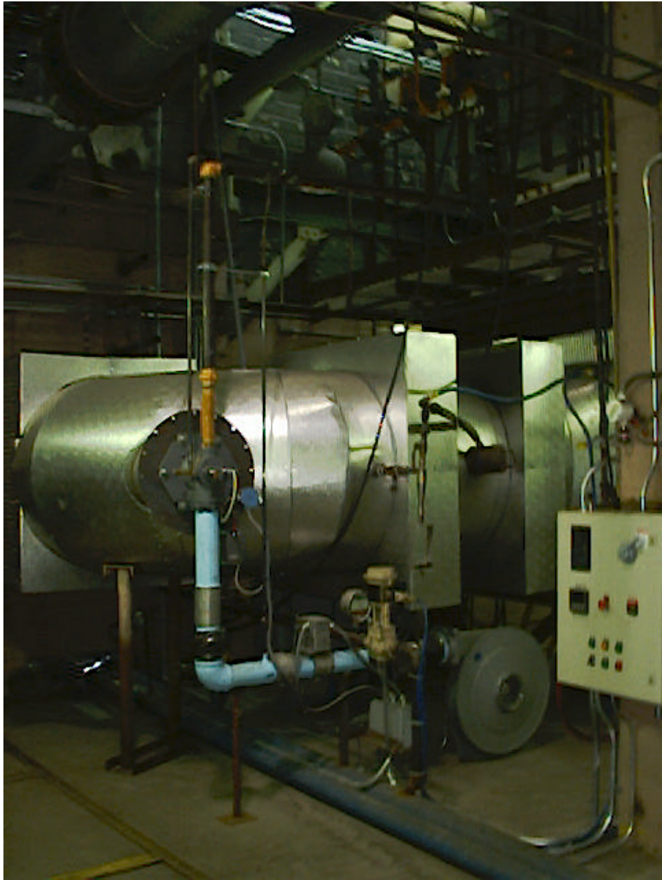
Figure 11 Reheat Burner
