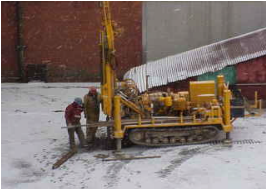
Figure 4. Geotechnical Investigations at the Willow Island Site
