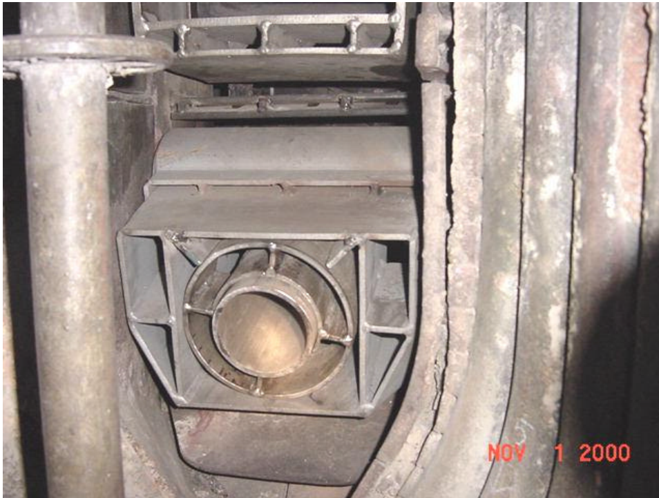
Figure 6. Installation of a Sawdust Nozzle at Albright Generating Station
