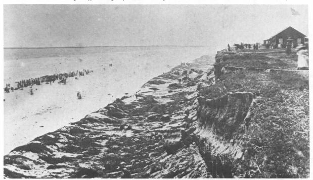
Figure 66. Summer 1885 photograph looking north along bluffs at Oceanside with wide beach below. Note: Extensive landslide material fronting the cliffs, showing predominance of subaerial erosion and lack of wave erosion (photograph from F. P. Shepard Collection).
