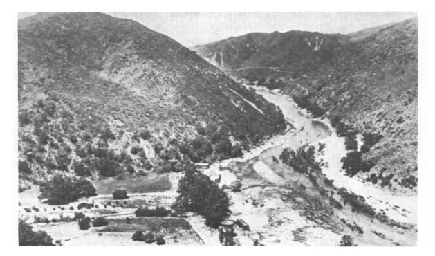
Figure 28B. View from same location as Fig. 28A in January 1916. Railway roadbed and bridges across the canyon were destroyed. Also note the occurrence of new landslides near the back of this photograph (photography from U.S. Geological Survey).
