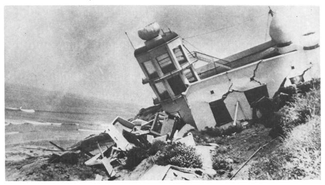
Figure 47b. View of temple collapse in the early 1940's following significant sea storms accompanied by saturation of the bluff top (photograph courtesy of Self Realization Fellowship).
