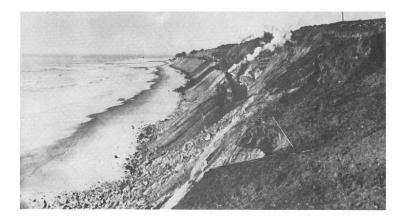
Figure 86. February 1910 view looking north along the cliffs at Del Mar showing construction of railroad bed (photograph by Santa Fe Railway Company).
