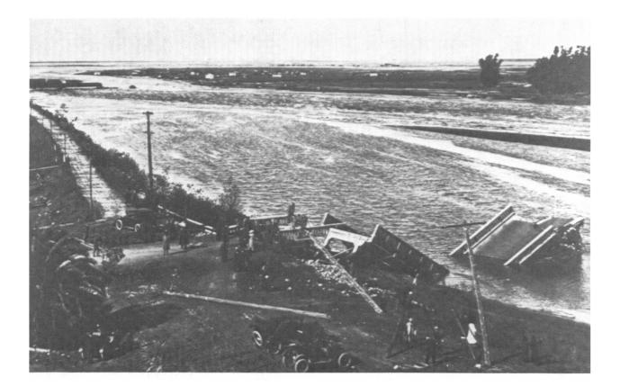
Figure 26. View looking west at bridge across San Diego River (Fig. 25) destroyed during flood in January 1916. All bridges across the San Diego River were destroyed during this flood (photograph from U.S. Geological Survey).
