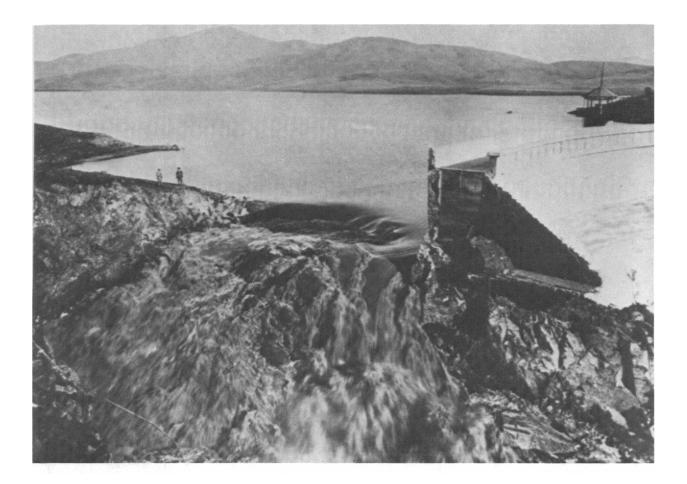
Figure 24. View across lateral break in Sweetwater Dam in January 1916 (photograph from U.S. Geological Survey).
