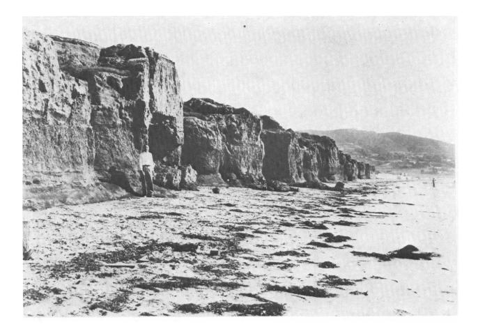
Figure 92. 1936 view of low-lying alluvial cliffs at Scripps. Cliffs were retreating at that time at a rate of about 1 foot per year (photograph by U.S. Grant IV).
