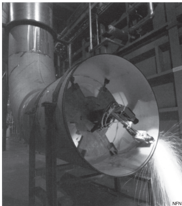
Figure 4. The Elbow Cutting Pipe Crawler was used to cut piping located 265 feet
