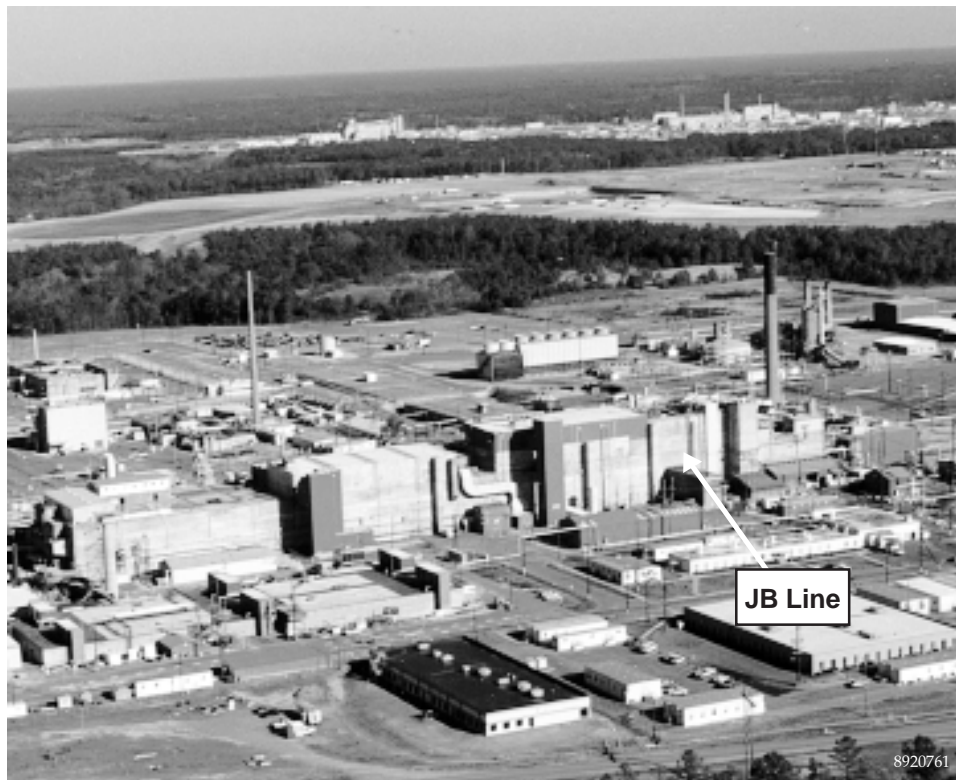
Figure 2. Building 221-F Canyon with JB-Line
