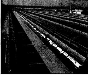
Nine trough power plants in California's Mojave Desert provide the world's largest generating capacity of solar electricity, with a combined output of 354 megawatts.
