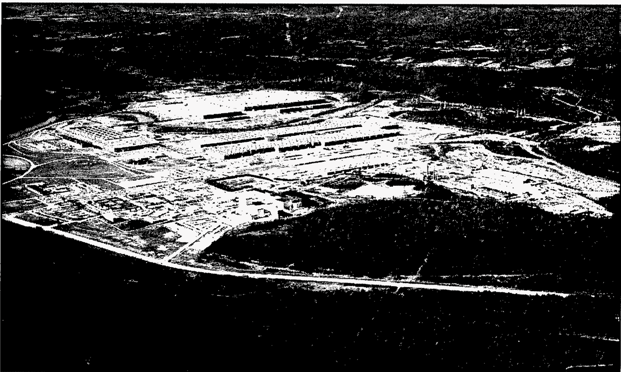
Fig. 1.6. The East Tennessee Technology Park (formerly the Oak Ridge K-25 Site).
