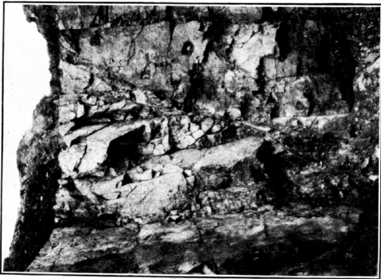
1. FACE OF EXCAVATION, SHOWING JOINTING.
