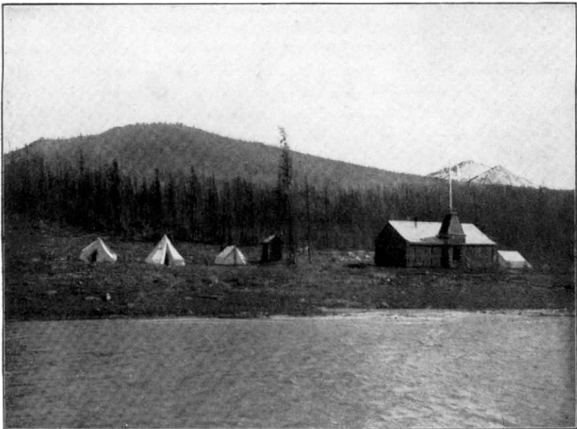
FIG. 2.—CANADIAN POLICE STATION AT CARIBOU CROSSING.
