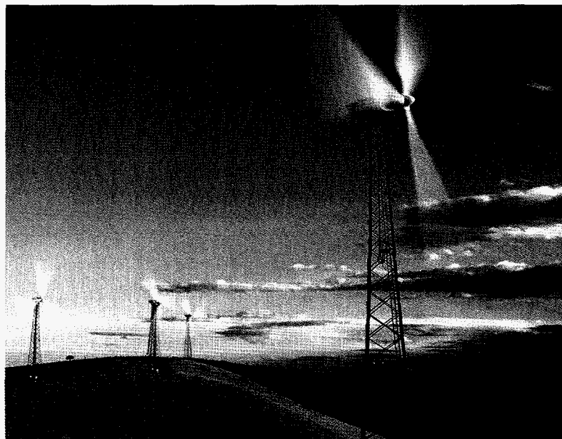
In the Great Plains, lightning can wreak havoc with wind turbines. Central and South West Services and Zond Systems, Inc., learned this lesson the hard way in Texas. The companies have since created state-of-the-art lightning protection systems for wind power plants.
