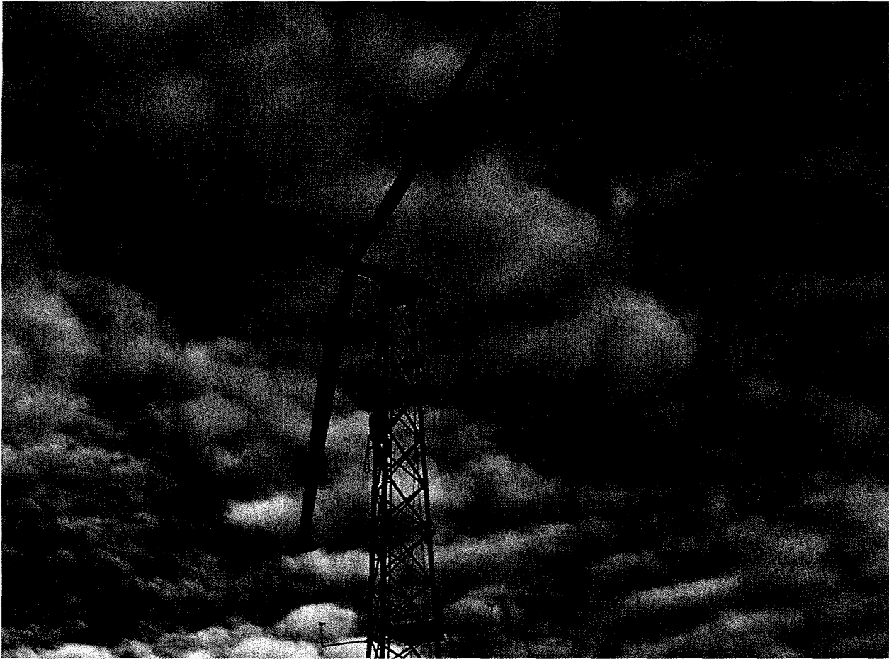
Kotzebue Electric Association operates a wind technology project north of the Arctic Circle in Alaska. The utility is participating in the turbine verification program's testing and evaluation efforts as an "associate" project. Associate projects receive funding from the program for performance evaluation only.
