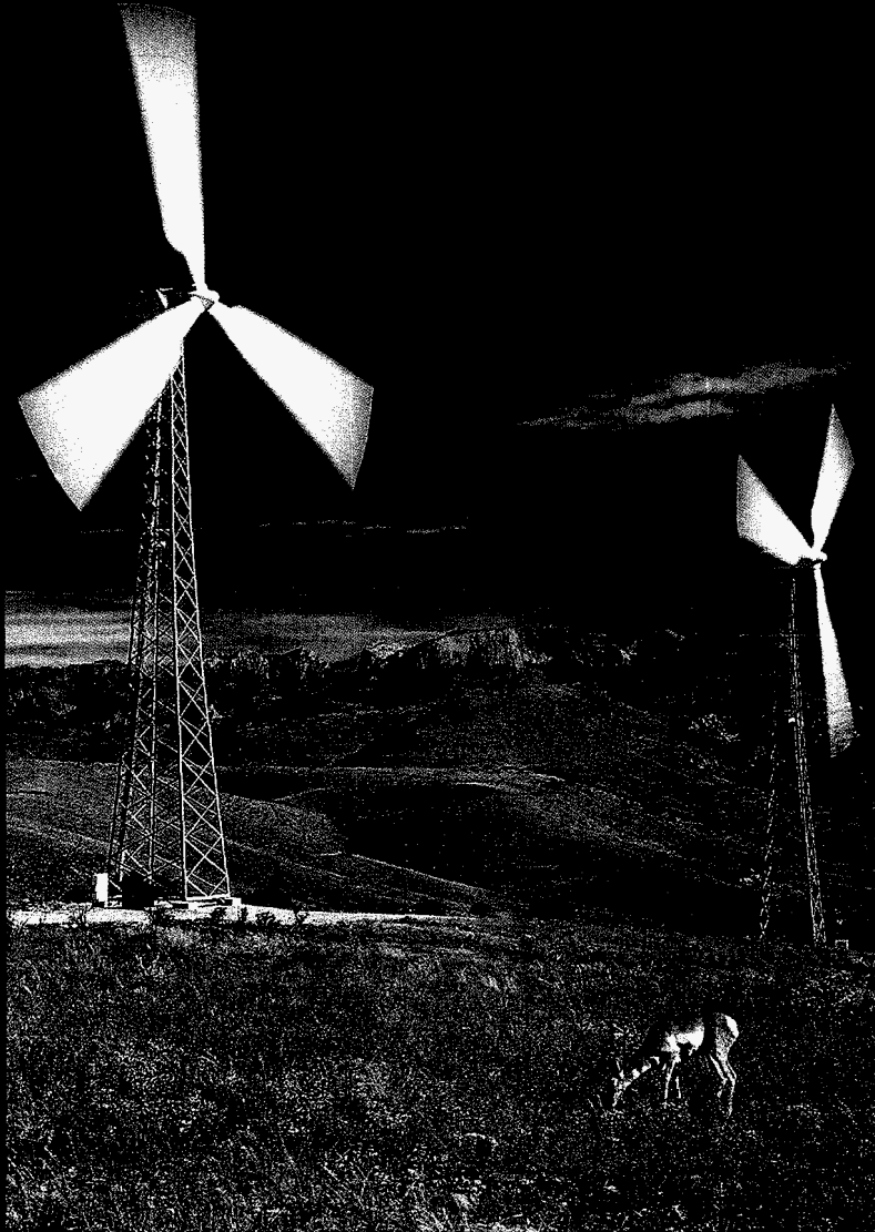
Central and South West Services, Inc., operates a 6.6-MW wind power plant in west Texas near Fort Davis. The facility was the first of its kind completed as part of the turbine verification program.
