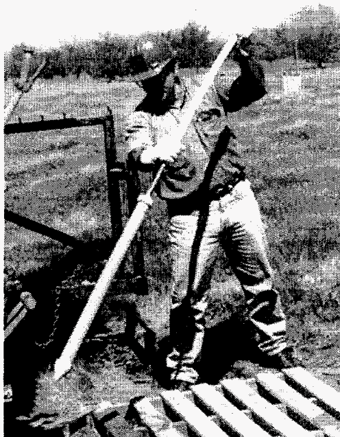
Figure 1. A flow sensor being installed through a hollow-stem auger.
