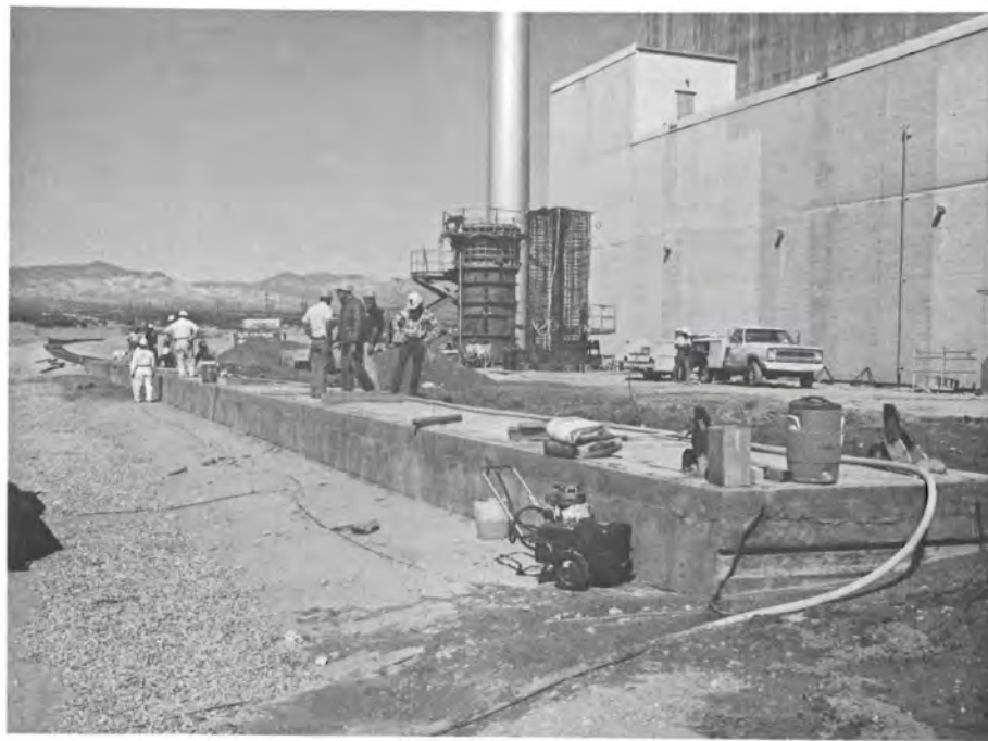
Figure B-13. Drywell Concrete Pad Construction Completed
