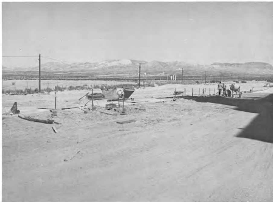
Figure B-16. Instrumentation Wells Installed in Drywell Storage Area
