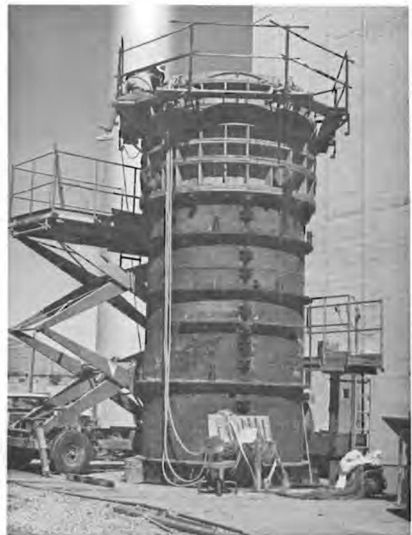
Figure B-21. Form for Concrete Silo Being Prepared for Concrete Pouring
