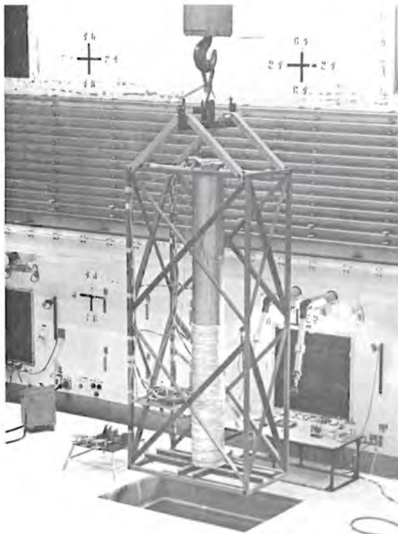
Figure B-67. Completed Test Assembly Being Lifted Prior to Transport to West Process Cell
