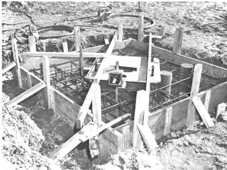
Figure B-4. Electrically Heated Drywell Pad Forming, Concrete Pouring Half Complete
