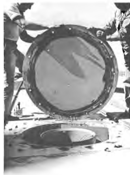
Figure 3.3-2. Drywell 3 Cover Plate Removed After Isolated Drywell Test Phase I
