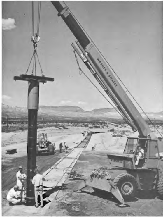
Figure B-14. Drywell Liner Installation Into Storage Area
