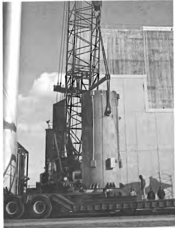
Figure B-23. Completed Concrete Silo (Shown During Dry Run of Handling and Operations)
