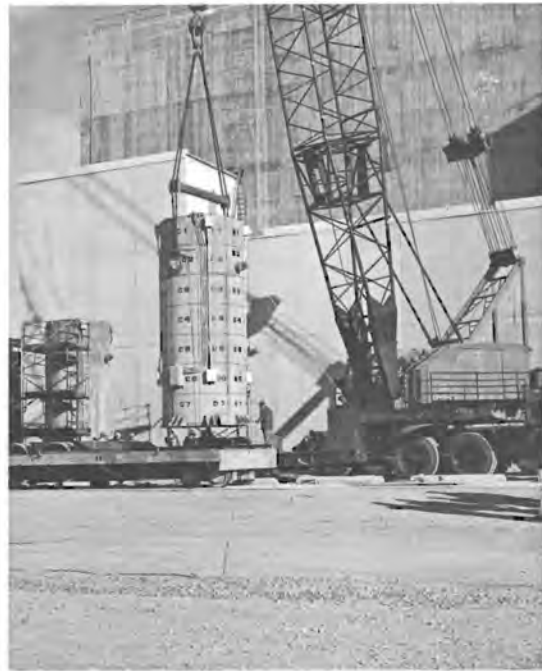
Figure B-61. Concrete Silo Transfer From Trailer to Storage Pad
