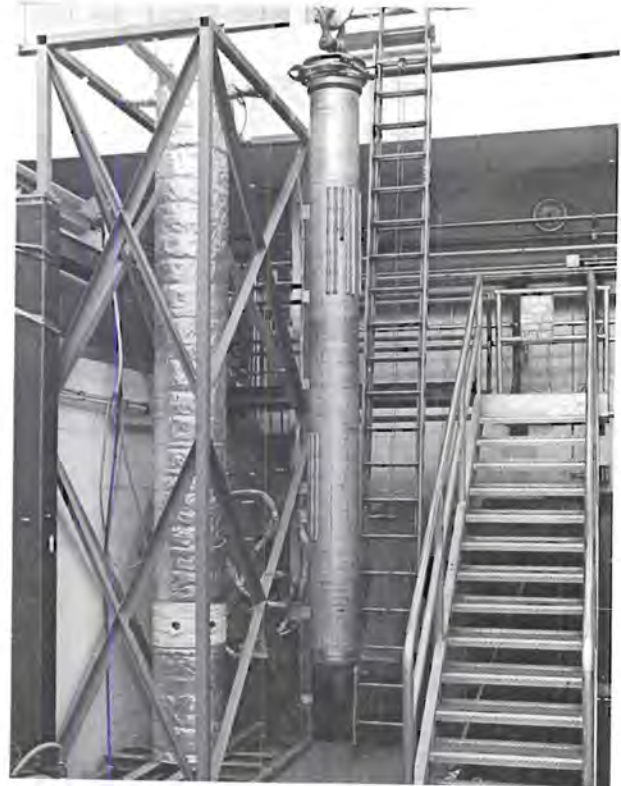
Figure 5.2-11. Completed Test Stand and Canister During Fitup Check
