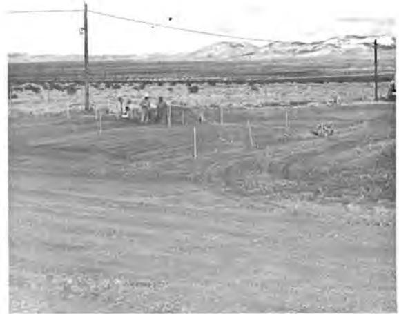
Figure B-3. Grading Completed for Electrically Heated Drywell
