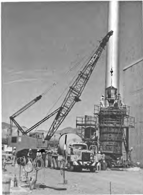
Figure B-22. Pouring of Concrete Into Form (Silo No. 2)
