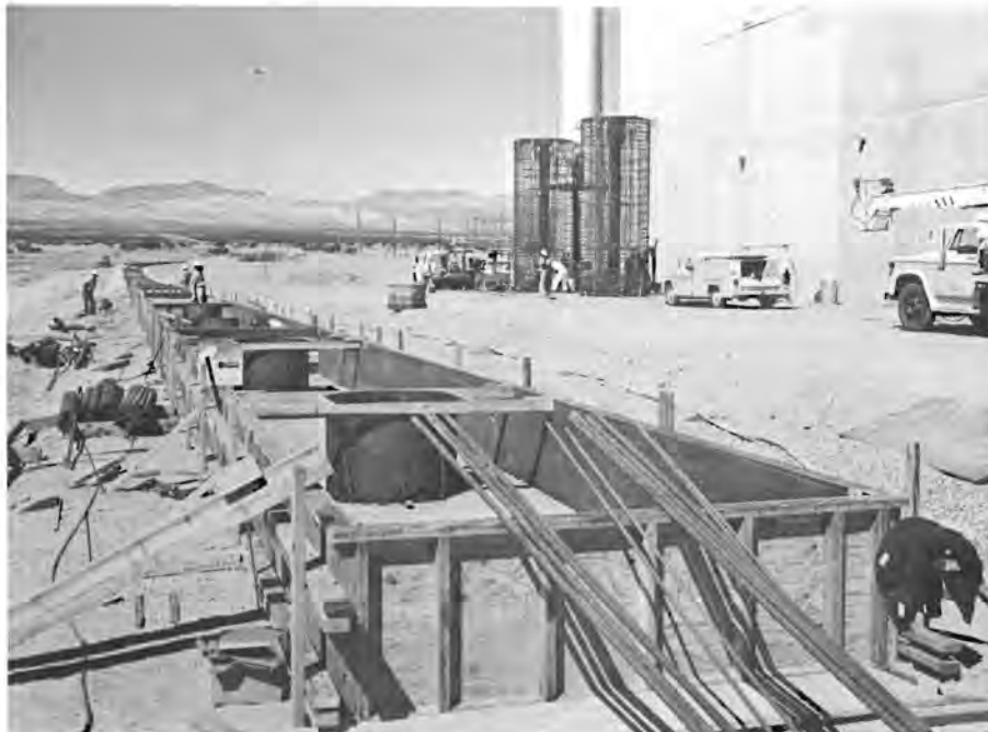
Figure B-11. Drywell Storage Area Construction
