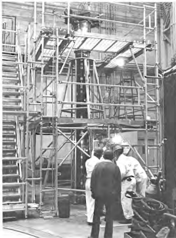
Figure 3.2-5. Thermocouples Installed on Liner
