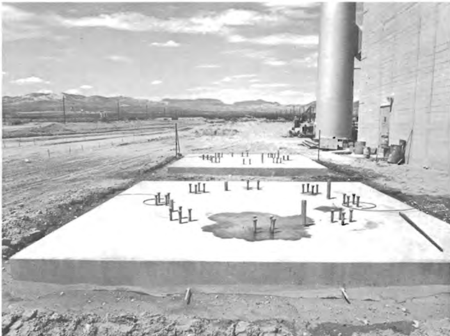
Figure B-19. Concrete Silo Support Pads-Construction Completed
