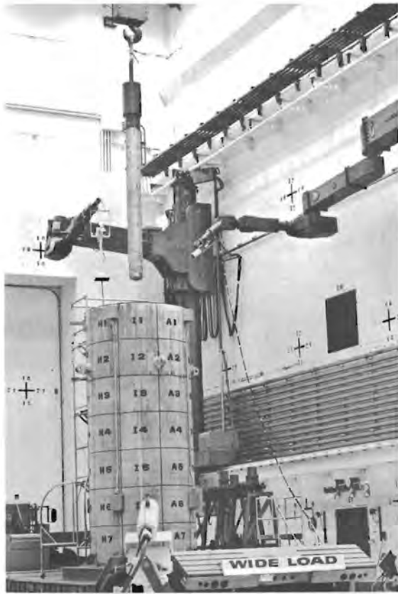
Figure B-60. Completed Canister Assembly Being Remotely Lowered Into Concrete Silo in Hot Bay
