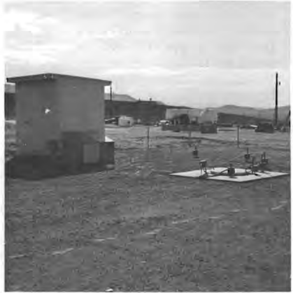
Figure B-9. View of Completed Electrically Heated Drywell
