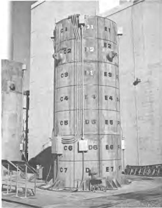
Figure 4.2-7. Completed Concrete Silo
