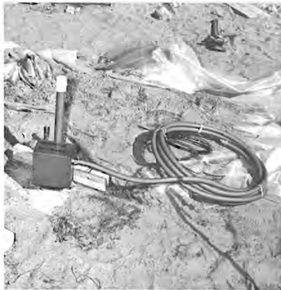
Figure B-7. Instrumentation Well Grouted in Hole
