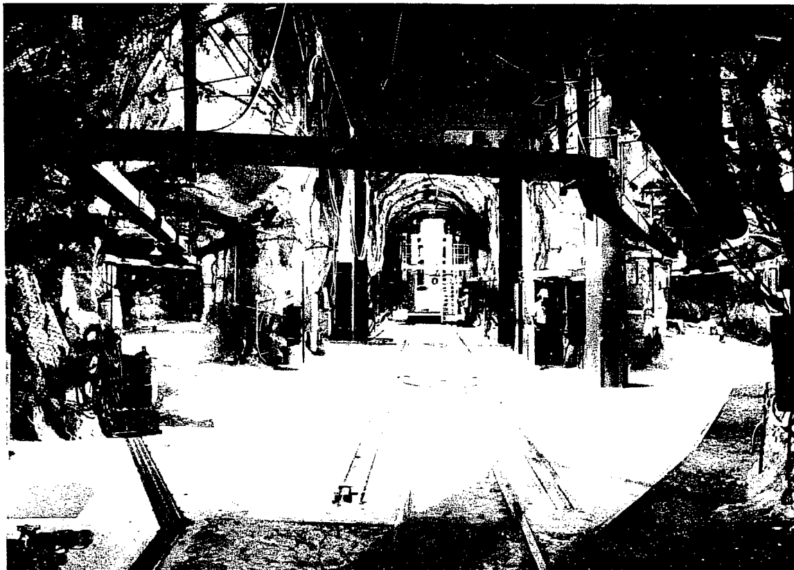
Figure 5-6. Panorama of Spent Fuel Test—Climax drifts.
