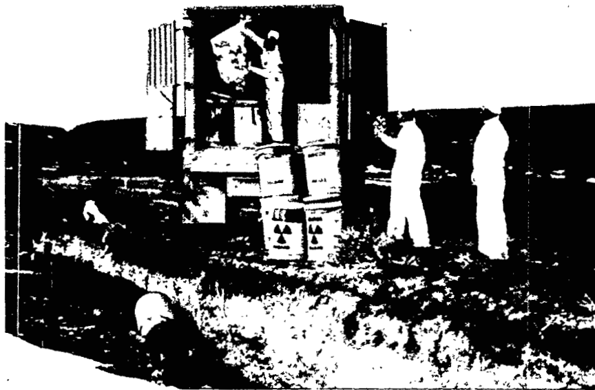
Low-level radioactive wastes being dumped into trenches for land burial at AEC's National Reactor Testing Center, Arco, Idaho. Man on truck wears protective clothing and respirator while man to his left monitors radiation. (Credit: National Archives)
