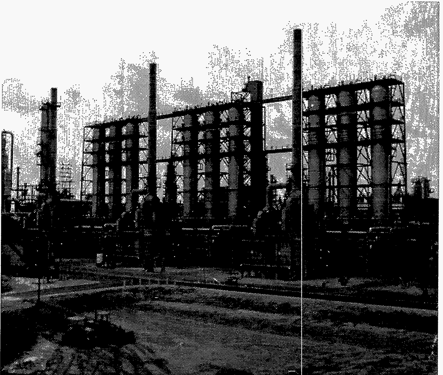
Downstream processing units are used to upgrade petroleum products.
