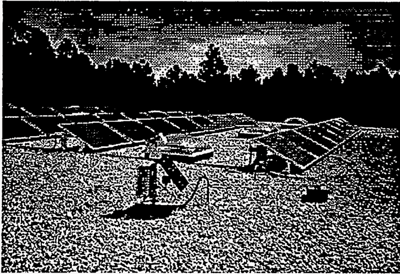
Figure 6. PV Array at INTEK, Inc.
