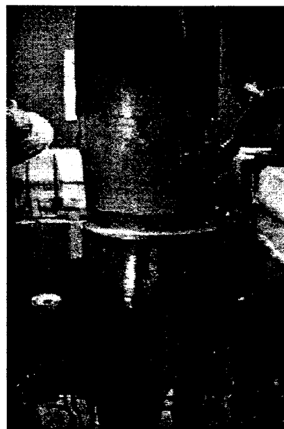
Figure 1 (left) shows the transfer cask being positioned to remove a fuel assembly from the reactor. The grapple can be seen sticking out just below the cask.
