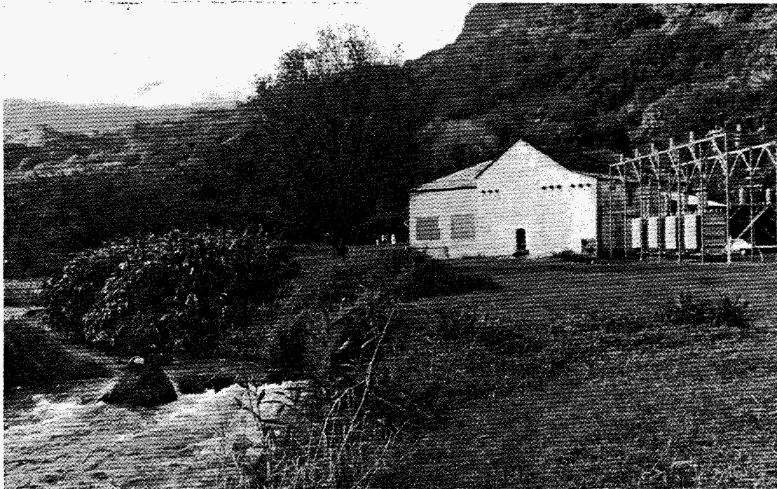
Figure 4. The Wainiha Hydroelectric Plant, on the Island of Kauai, is an example of a developed site in Hawaii. The Wainiha plant, located on the Wainiha River, has a nameplate capacity of 3,600 kW and it produces an average of 24 million kWh of electricity annually. The plant has a gross hydraulic head of 560 feet and it has an average inflow of about 80 cubic feet per second of water.
