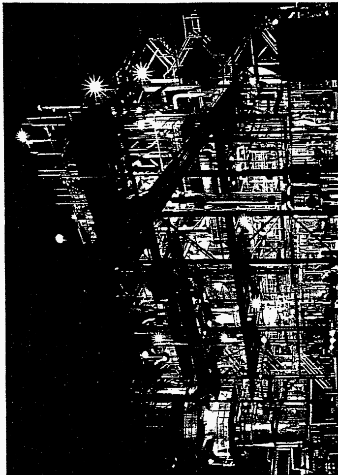
Hercules' production site at Brunswick, Ga., is one of the company's primary rosin resin plants.
