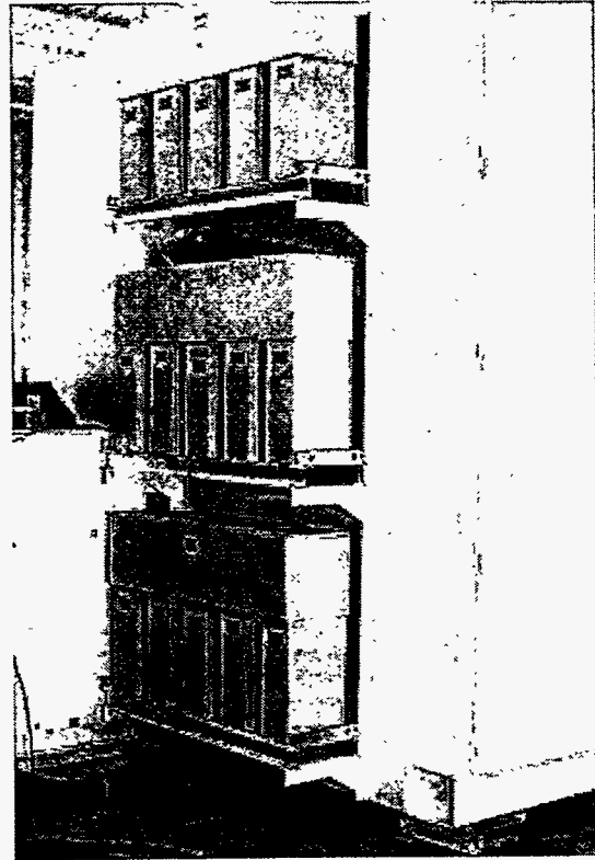
Figure 7. AC Battery System Container with "Cap Banks"
