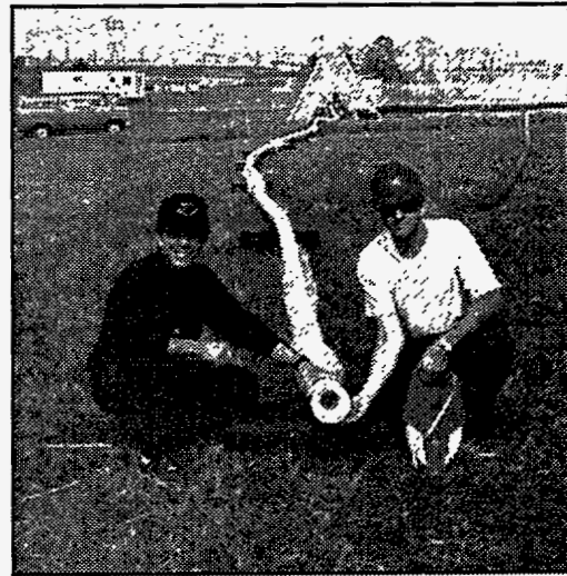
Figure 1.5-2. Microporous Pipe Used in Construction of Recirculation Wells.
