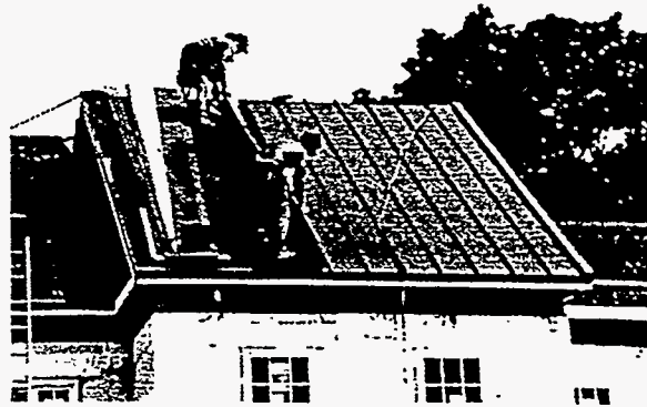
Figure 14 Placement of Metal Roofing Panel
