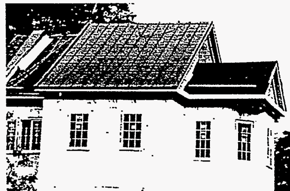
Figure 18 12 Panels Installed on Middle Section
