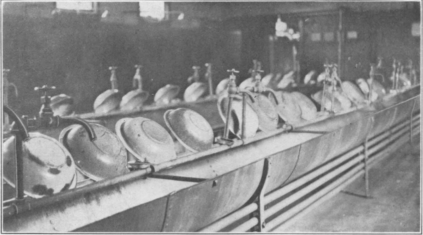
A. A SEMICIRCULAR WASH TROUGH WITH BASINS IN DRYING POSITION.
