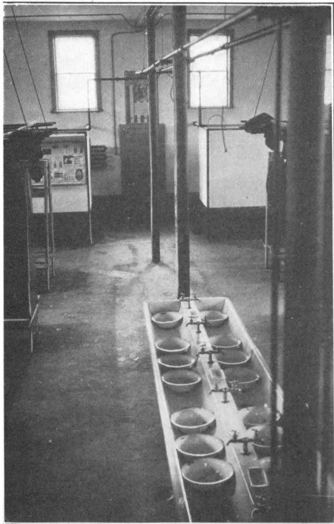
A. A DOUBLE TROUGH OF WHITE ENAMELED IRON EQUIPPED WITH BASINS. NOTE BULLETINS IN THE REAR.
