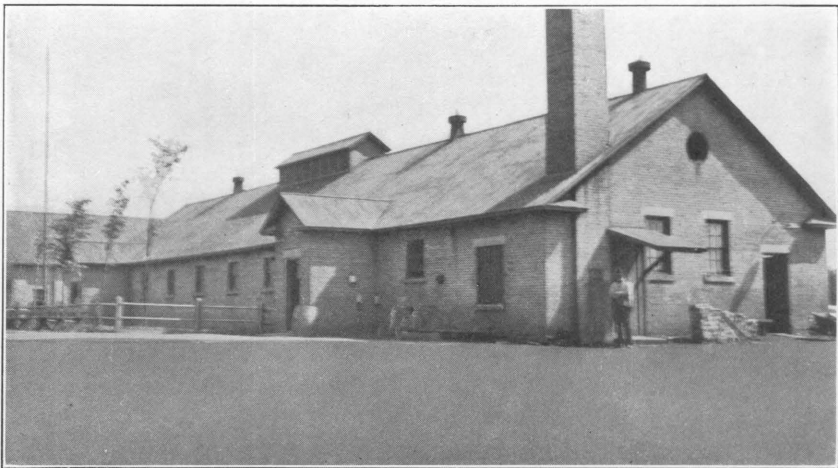
B. A CHANGE HOUSE OF BRICK WITH A CORRUGATED-IRON ROOF. LONG WOODEN VENTILATING MONITOR AND SMALL VENTILATORS OF SHEET IRON.
