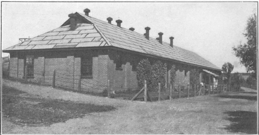
B. A BRICK CHANGE HOUSE WITH A RUBBEROID ROOF AND SANITARY SURROUNDINGS.
