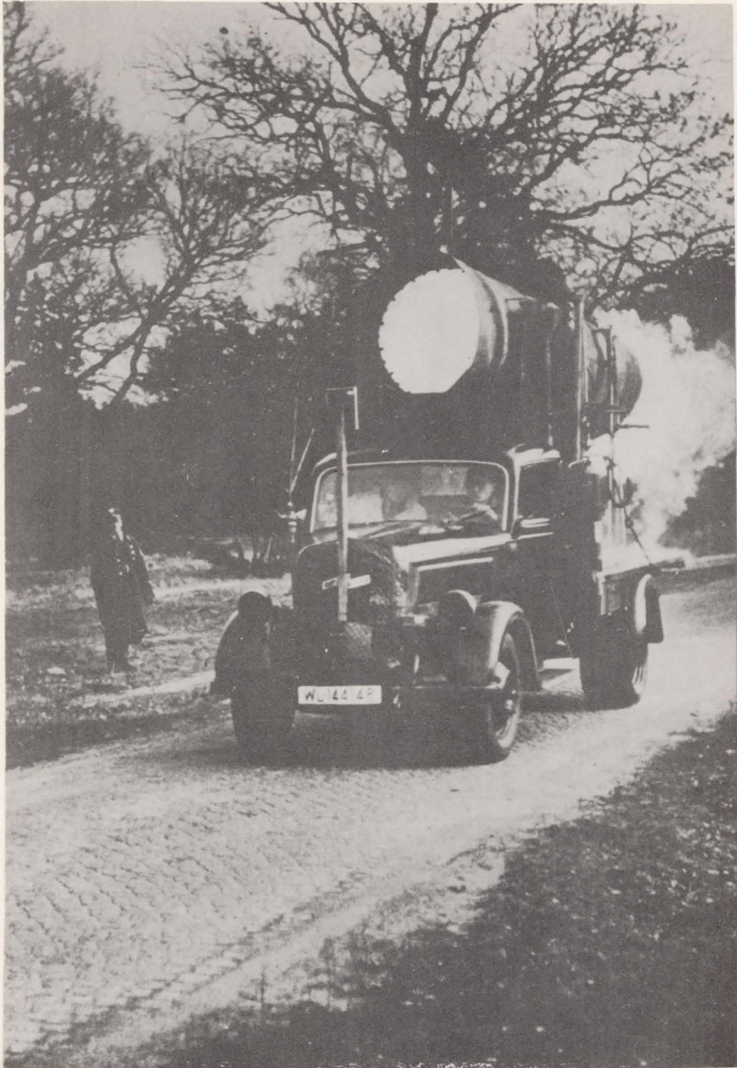
Figure 19.- Road towing test with Lorin combustion chamber of 800-mm diameter and 2400°K discharge temperature for studying the injection and combustion processes.
