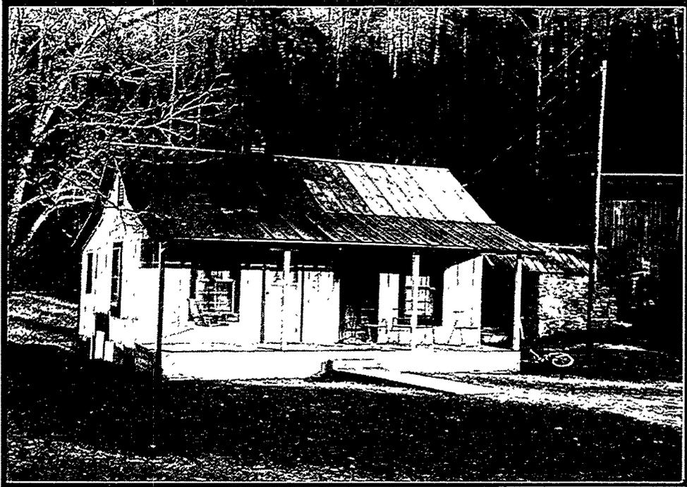
Figure 10: The Grayson House is a saddlebag plan example of boxed construction.
