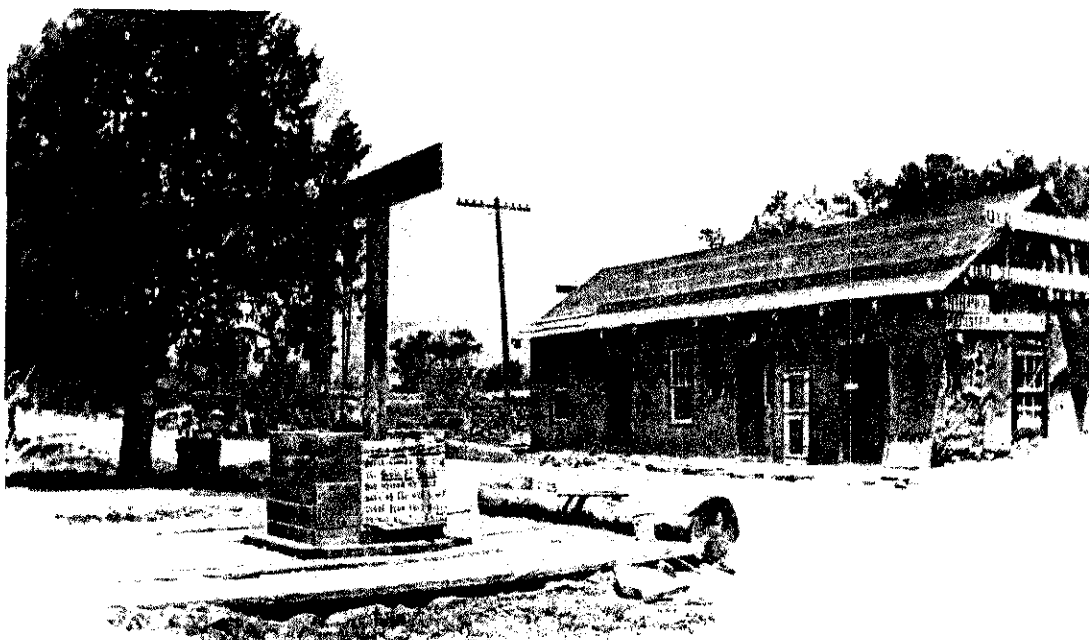
Figure 8: Pigeon's Ranch, ca. 1925. Building is more like it appears today. Image #51738 at Photo Archives, Museum of New Mexico, Santa Fe, NM.
