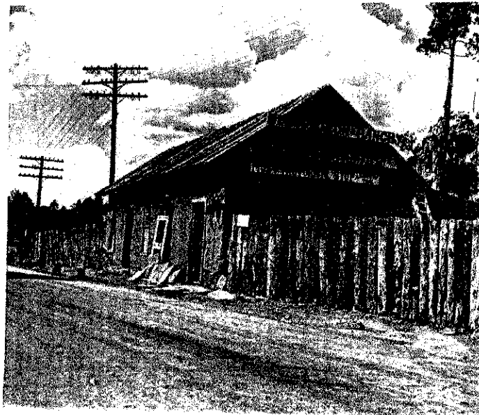
Figure 13: Pigeon's Ranch showing deterioration over the years, ca. August 1951. Image #90717 at Photo Archives, Museum of New Mexico, Santa Fe, NM.
