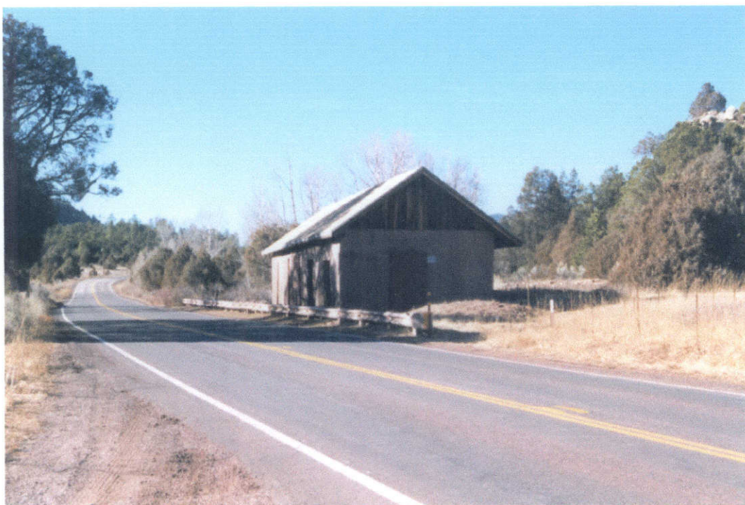
Figure 19: The Pigeon's Ranch building with guard rail as sole protection against an errant driver. Photo by author.
