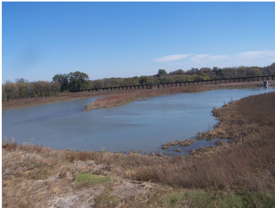
Figure 1.12. Aquatic vegetation establishment in the DFE LCOW's developing wetland cell E
