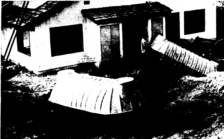
Figure XI-4.— Installation of Fiberglass Underground Tanks
