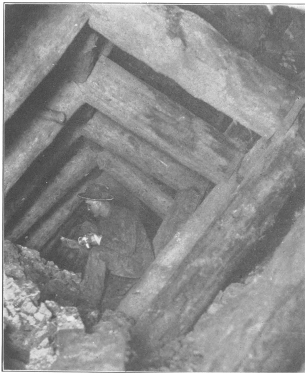
B. FOUR-PIECE SET ROCKER FRAMING IN NARROW INCLINED VEIN.
