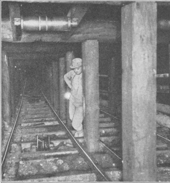
A. VIEW OF THE TIMBERING EMPLOYED IN SHAFTS INCLINED LESS THAN 30^{\circ} . NOTE THE ROLLER AT THE TOP OF THE SHAFT AND THE DIVIDING POSTS BETWEEN THE TWO COMPARTMENTS.
