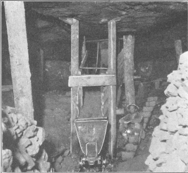
A. CHUTE AND CAR USED IN THE STULL METHOD OF STOPE TIMBERING.
