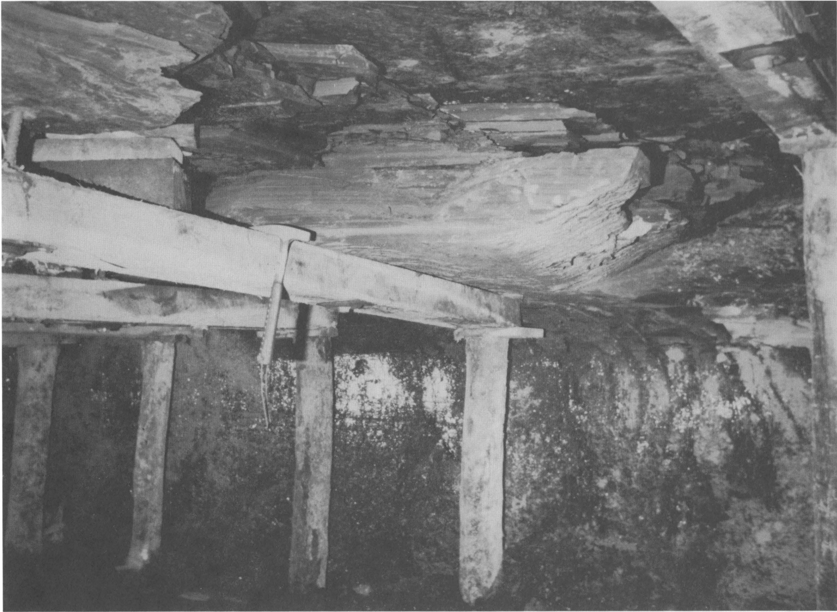
FIGURE 16. - Photograph of horizontal slickensided plane within shale roof-rock of the main entries.
