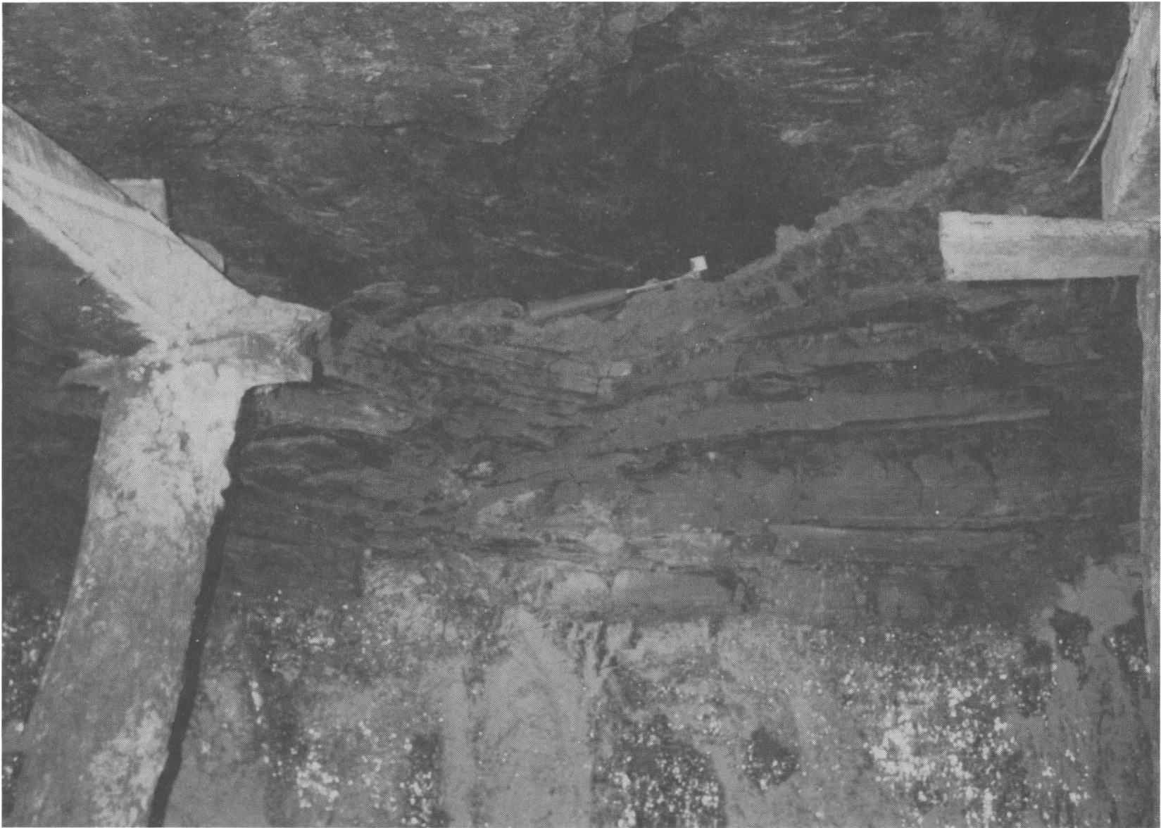
FIGURE 25. - Photograph of the bedding plane fault associated with thrust faults. Notice the horizontal slickensided plane and fault gouge.
