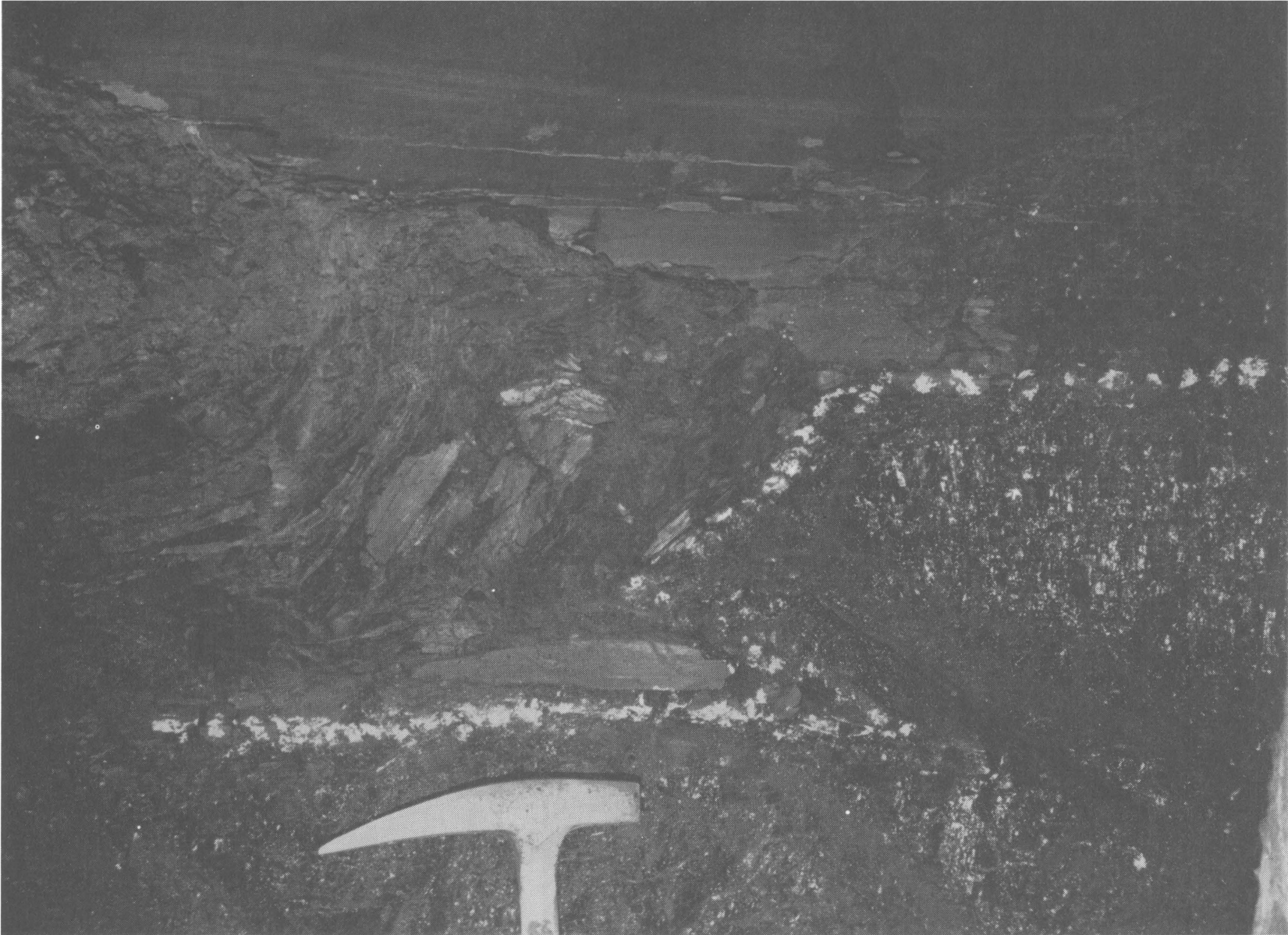
FIGURE 19. - Photograph of thrust fault with structurally disturbed coal and shale roof-rock.
