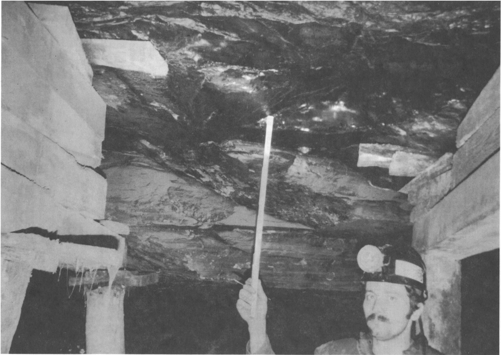
FIGURE 14. - Photograph of small, high-frequency, randomly oriented, slickensided planes in the transition zone of the study mine.
