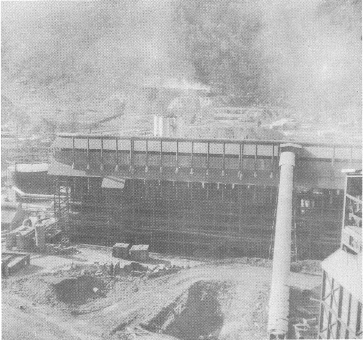
Figure 14. - Showing No. 11 conveyor from storage bins, lower right, to retorts.
