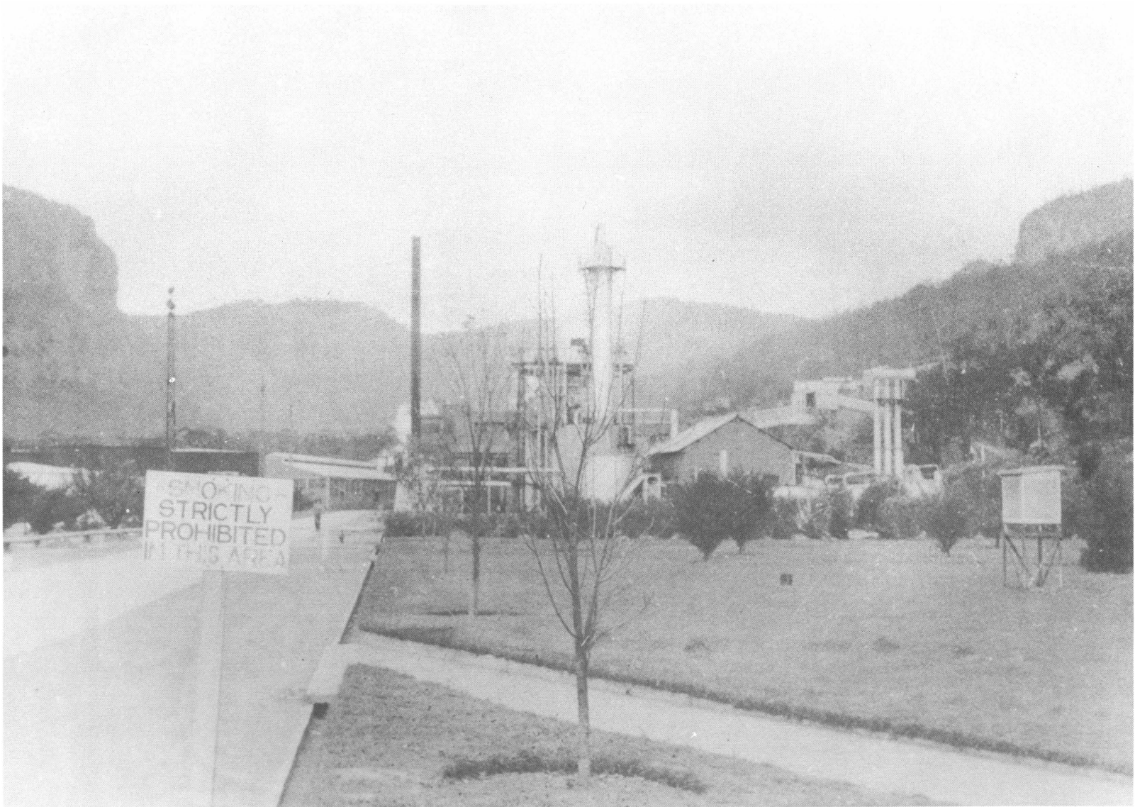
Figure 21. - National Oil Proprietary, Ltd., oil-shale plant, Glen Davis, N. S. W., Australia. Refinery in background.
