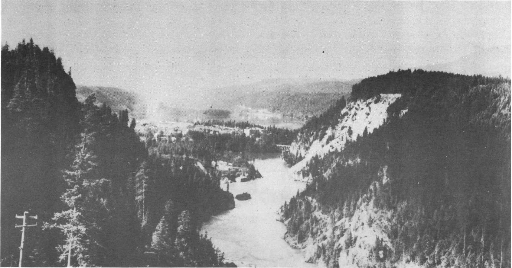
Figure 1. - Looking south from Grandview mine showing Pend Oreille power plant, Metaline Falls on the Pend Oreille River, the town of Metaline Falls, and the Metaline mine in the distance.
