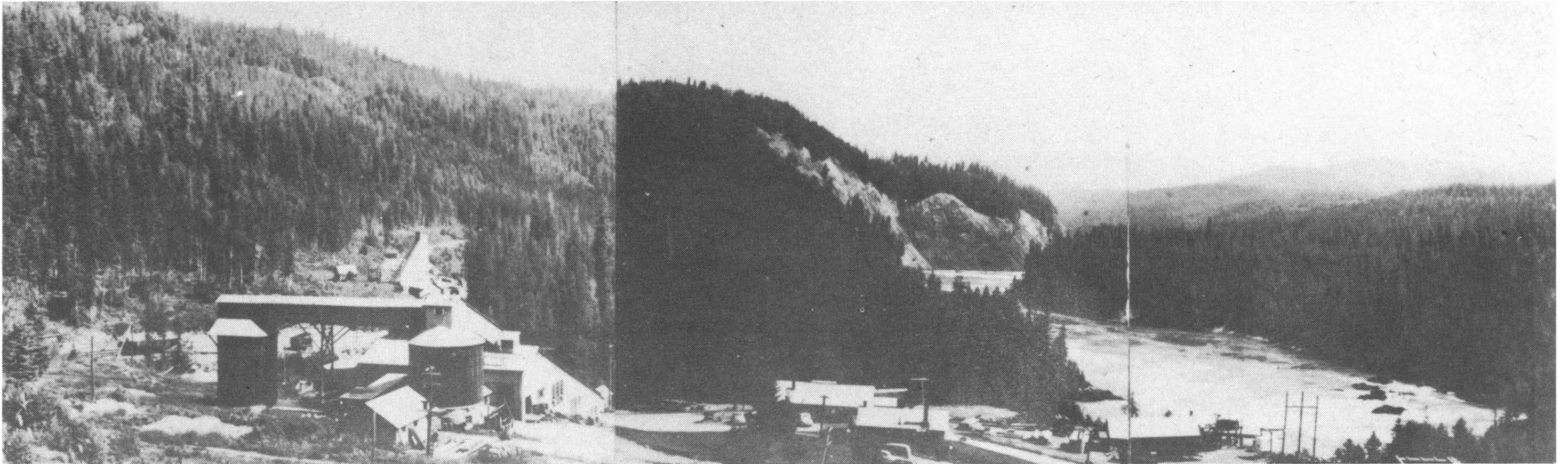
Figure 2. - View showing Pend Oreille mill, No. 1 shaft, Josephine mine, and Pend Oreille River. Slate Creek Canyon in center background.
