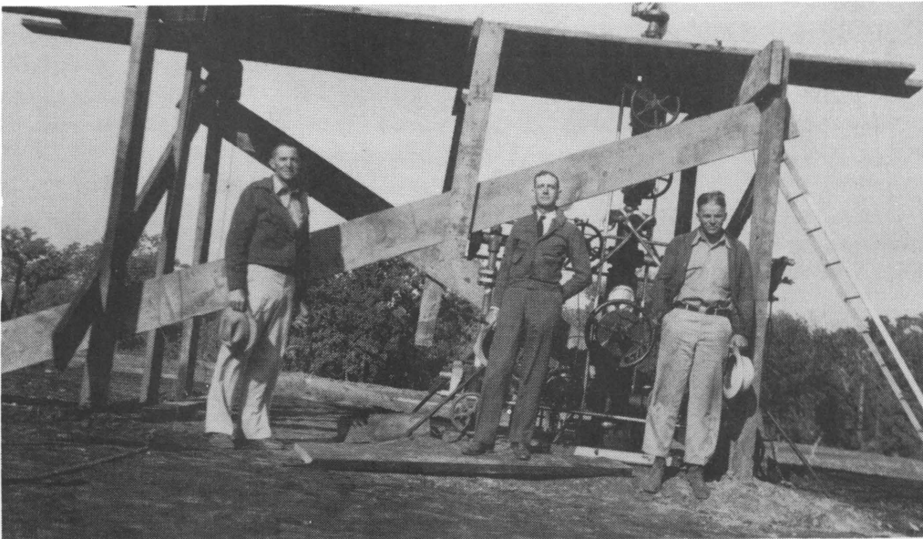
Figure 2.- Wellhead "Christmas tree."
