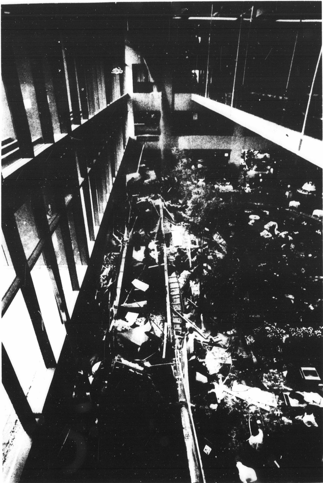
Figure 4.2 Walkways shortly after the collapse. View is directly to the north along the axis of the walkways. Span U7-8 is in foreground and third floor walkway is at upper right. Water is coming from broken sprinkler pipes. Photo by Greg Smith, reprinted by permission of The Kansas City Times , © 1981, The Kansas City Star Company.
