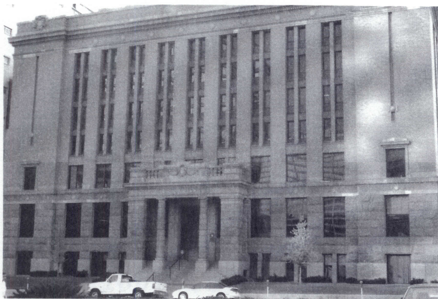
Figure 17: Tarrant County Criminal Courts Building
