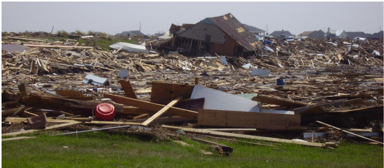
Figure 29. Flooding destroyed this home on Pontchartrain Drive in southern Slidell. Photo taken by Tisha Slagle, September 17, 2005.
