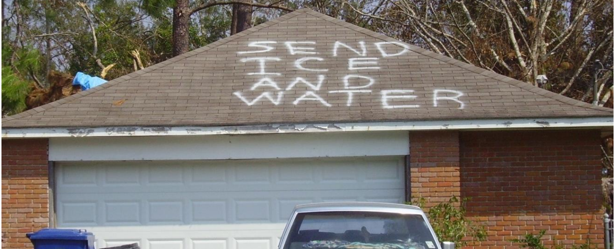
Figure 42. Sign spray-painted in white on the roof of a central Slidell home with a message to SEND ICE AND WATER. Photo taken by Tisha Slagle, September 16, 2005.
