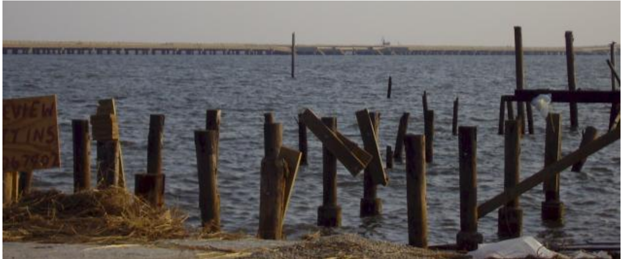
Figure 9: Remains of lakehome swept away by surge in southern Slidell. Photo taken by Tisha Slagle, September 17, 2005.
