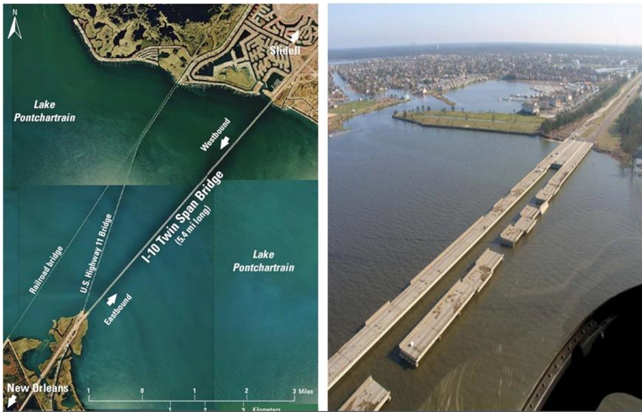
Figure 8. The Interstate 10 Twin Span bridges Slidell and New Orleans. Concrete segments of the bridge were twisted and many other segments washed away entirely by Katrina. Map from Google maps; photo from www.nola.com .
