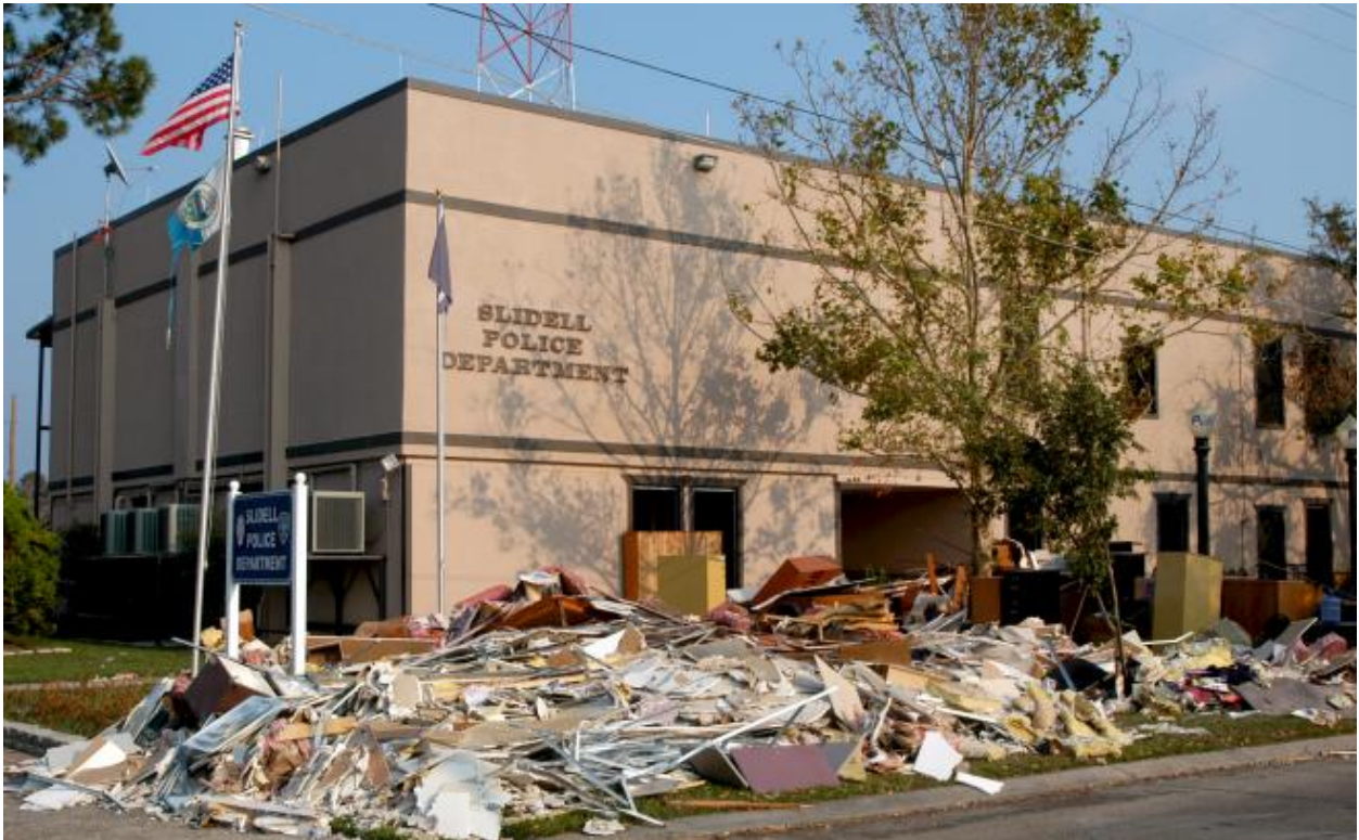
Figure 24. Flood-damaged debris from the interior of the Slidell Police Station. From http://www.slidell.la.us .
