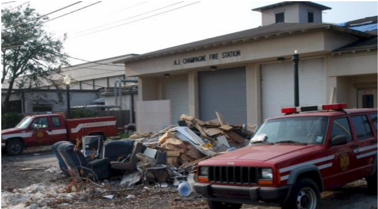
Figure 25. Flood-damaged debris removed from building and piled in front of Slidell's Fire Station. From http://www.slidell.la.us .
