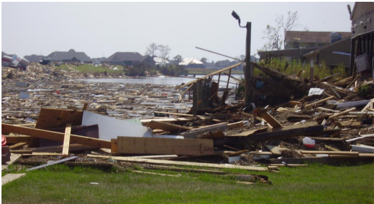
Figure 10. Debris from homes in south Slidell. Photo taken by Tisha Slagle, September 17, 2005.
