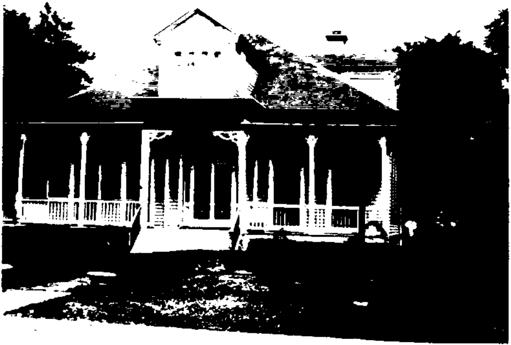
Figure 173. McKanara House Exterior.
