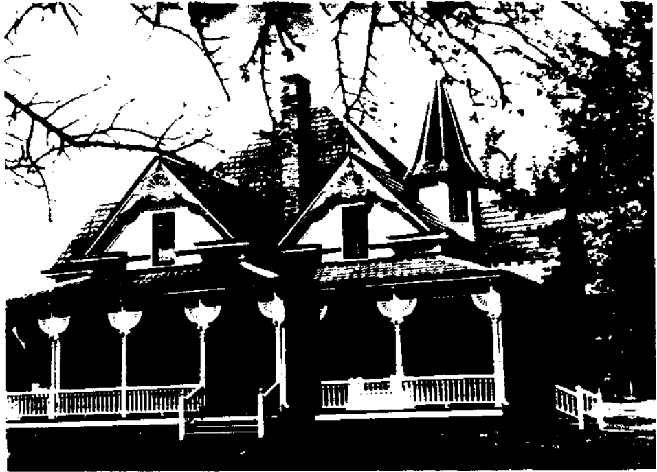
Figure 142. George House Exterior.
