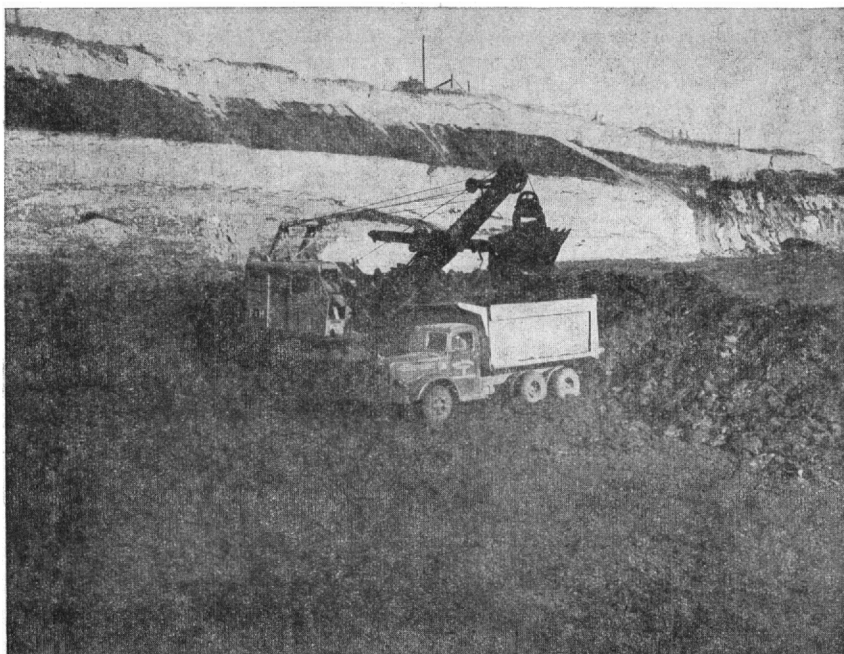
LOADING LIGNITE FROM THE LOWER BENCH OF THE HARMON BED AT THE PEERLESS MINE View northeast in sec. 34, T. 131 N., R. 99 W., Bowman County, N. Dak. The weathered upper bench is about 7 feet thick and is separated from the main bench of the Harmon bed by about 15 feet of clay.
