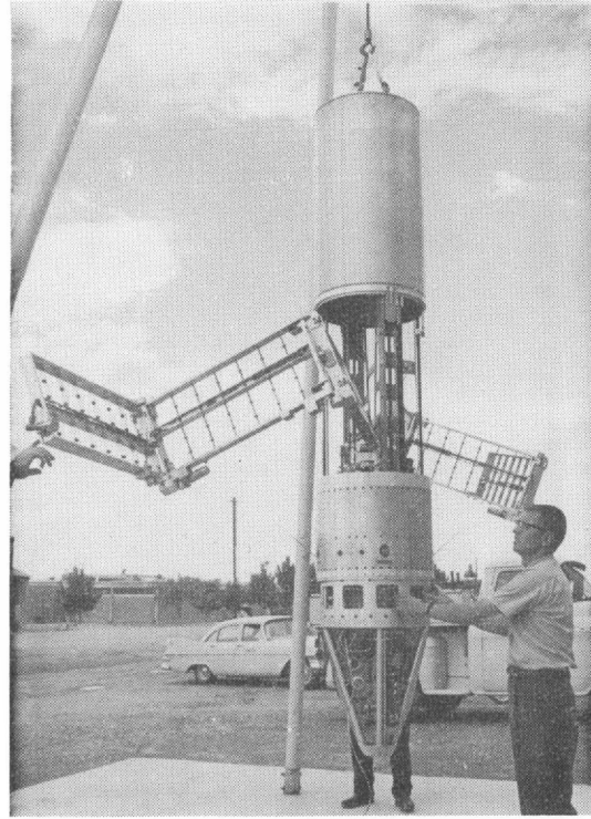
Figure 95. SAND-LO rocket sampler-- blades being extended
