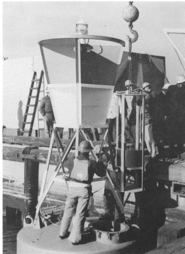
Fig. B-21. Battery and Converter Compartment Is Lowered into Light Buoy After Launching
