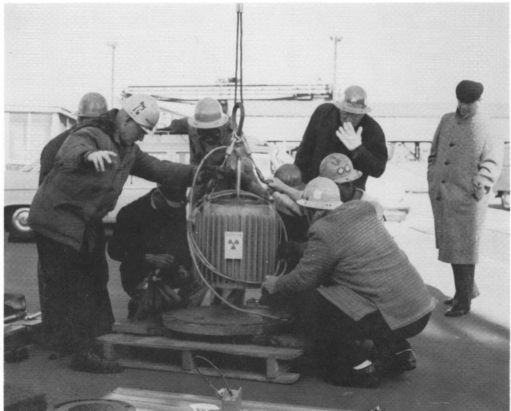
Fig. B-15. Generator Is Lowered onto Steel Flange and Loading Fixture
