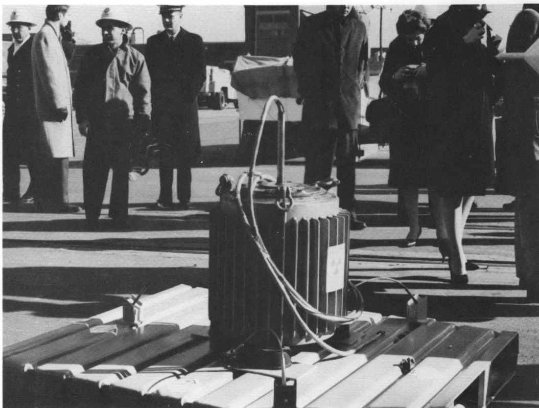
Fig. B-12. Generator Is Released from Shipping Pallet Restraining Cables
