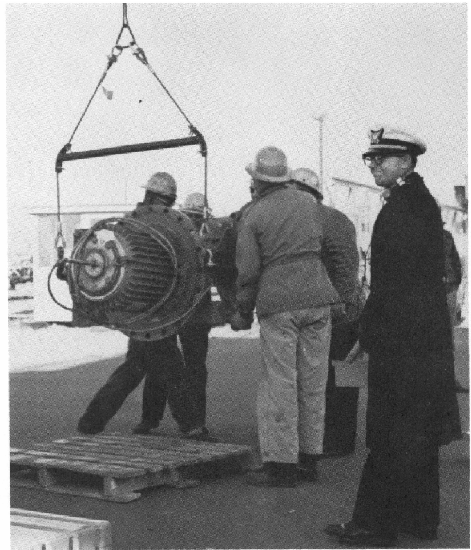
Fig. B-17. Generator Is Tilted to the Horizontal Position by Loading Fixture
