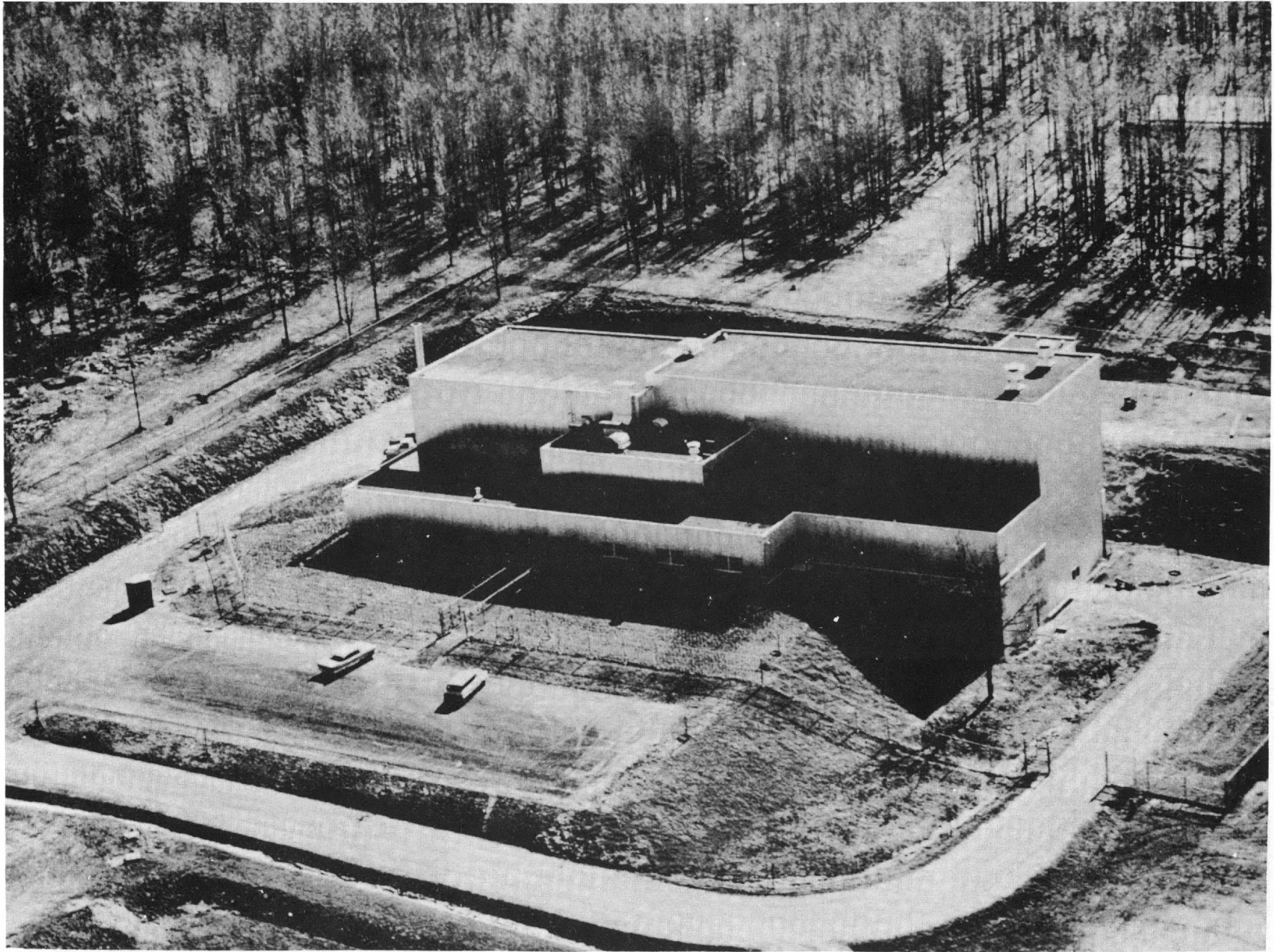
Fig. A-4. Exterior View of Laboratory Building
