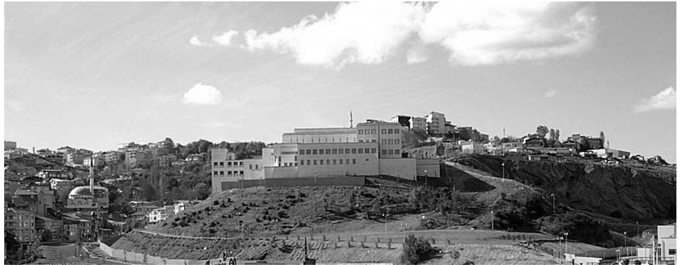
Figure 4: Consulate Building under Construction in Istanbul, Turkey
